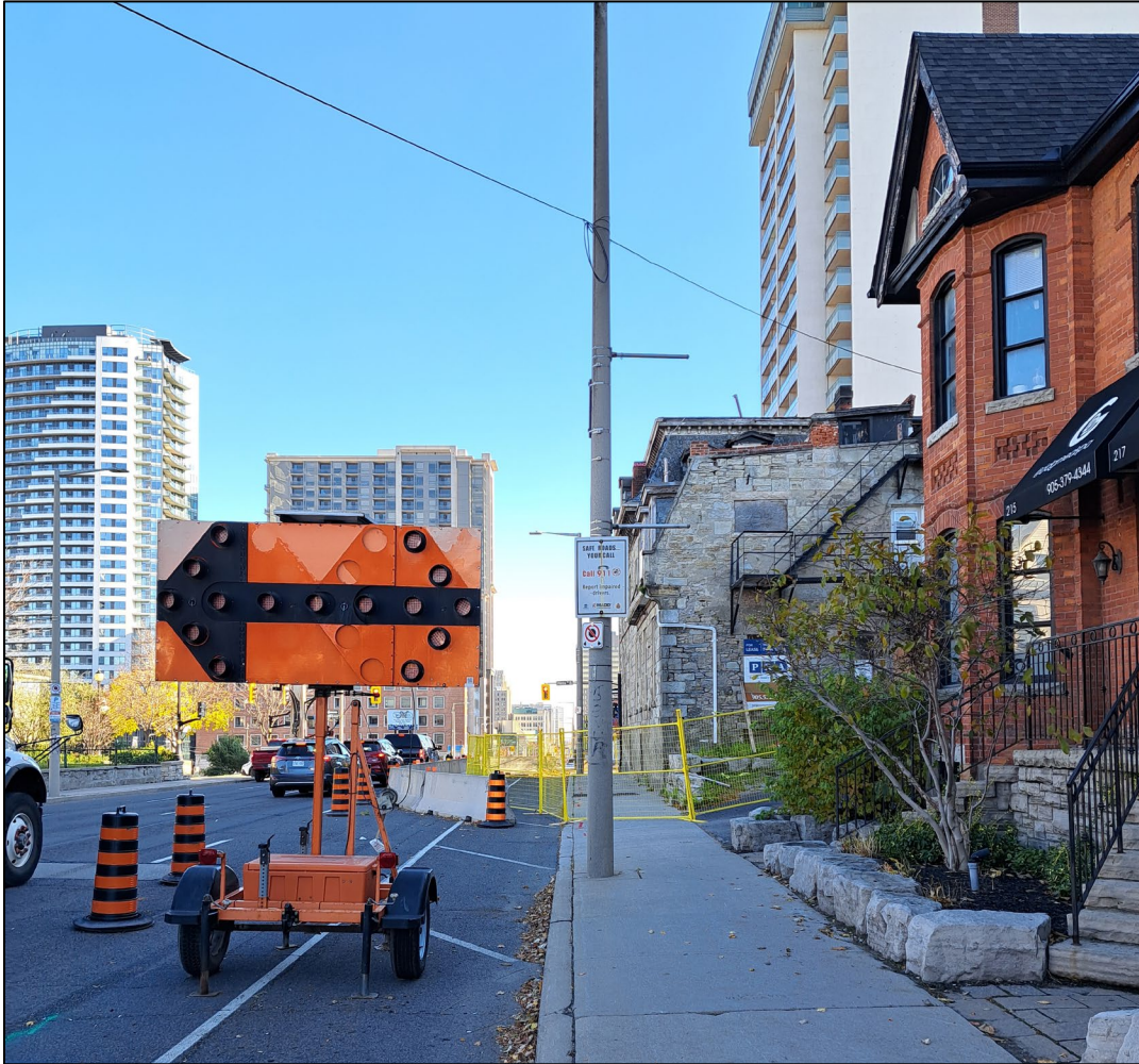
Closure of adjacent sidewalk and one lane of Main Street West
