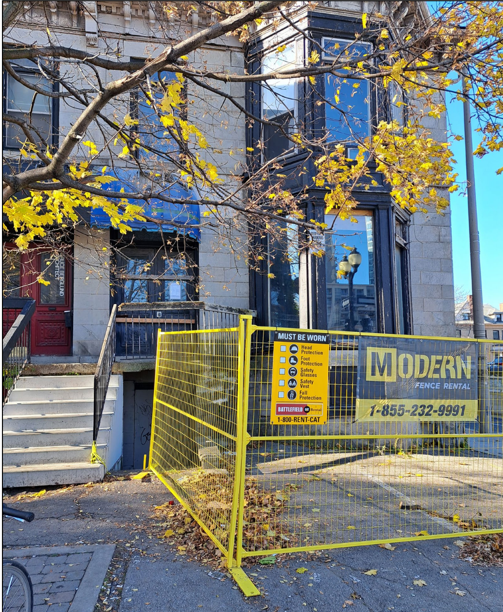
Front (east) elevation of 54 Hess Street South showing the safety fencing in place
