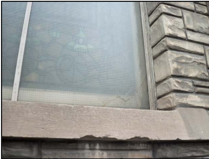
Photo No. 19: Cracked Windows
