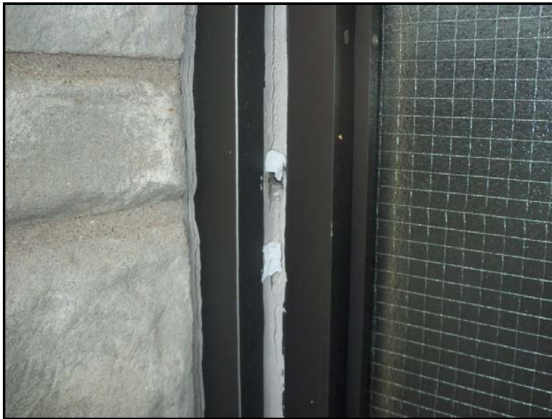
Photo No. 24: Deteriorated Sealant
