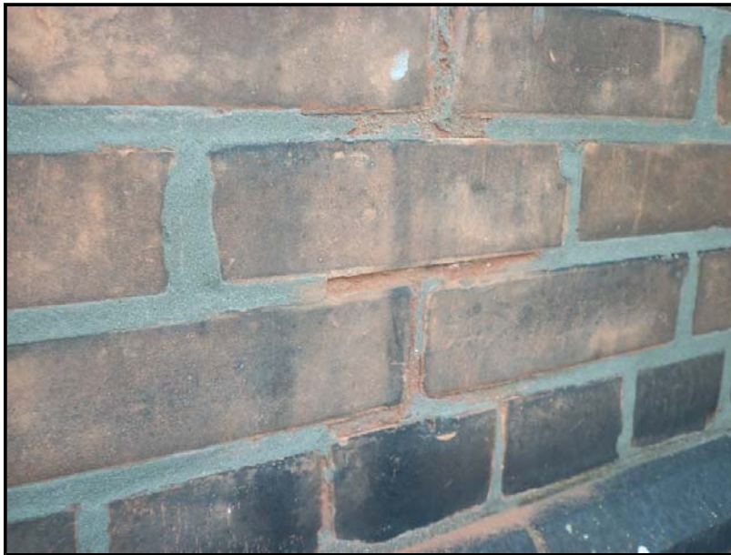
Photo No. 23: Deteriorated Mortar
