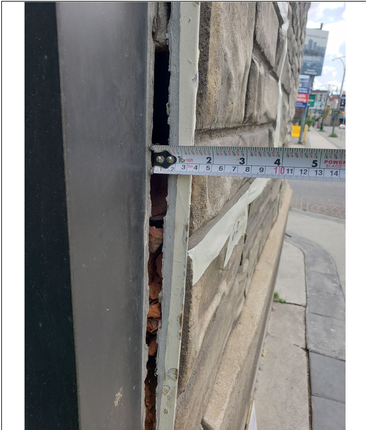
Photograph No. 23, showing a side view of the stonework for Exploratory Opening No. 2, adjacent to the door, prior to removal of the stone. Note the separation of the stonework to the brickwork, and visible freeze-thaw damage to the brick.
