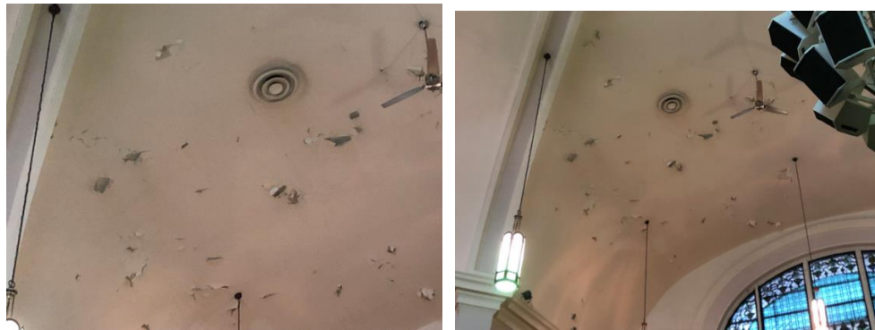
Figure 1: View of typical damage on Sanctuary ceiling
