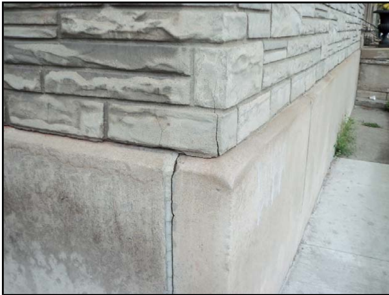
Photo No. 21: Cracks in Cementious Wall
