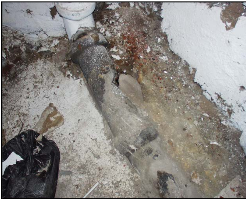
Photo No. 40: Broken Drain Pipe
