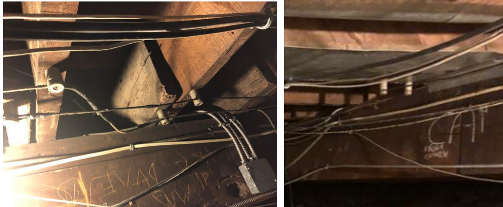
Figure 15: Examples of knob and tube wiring in basement
