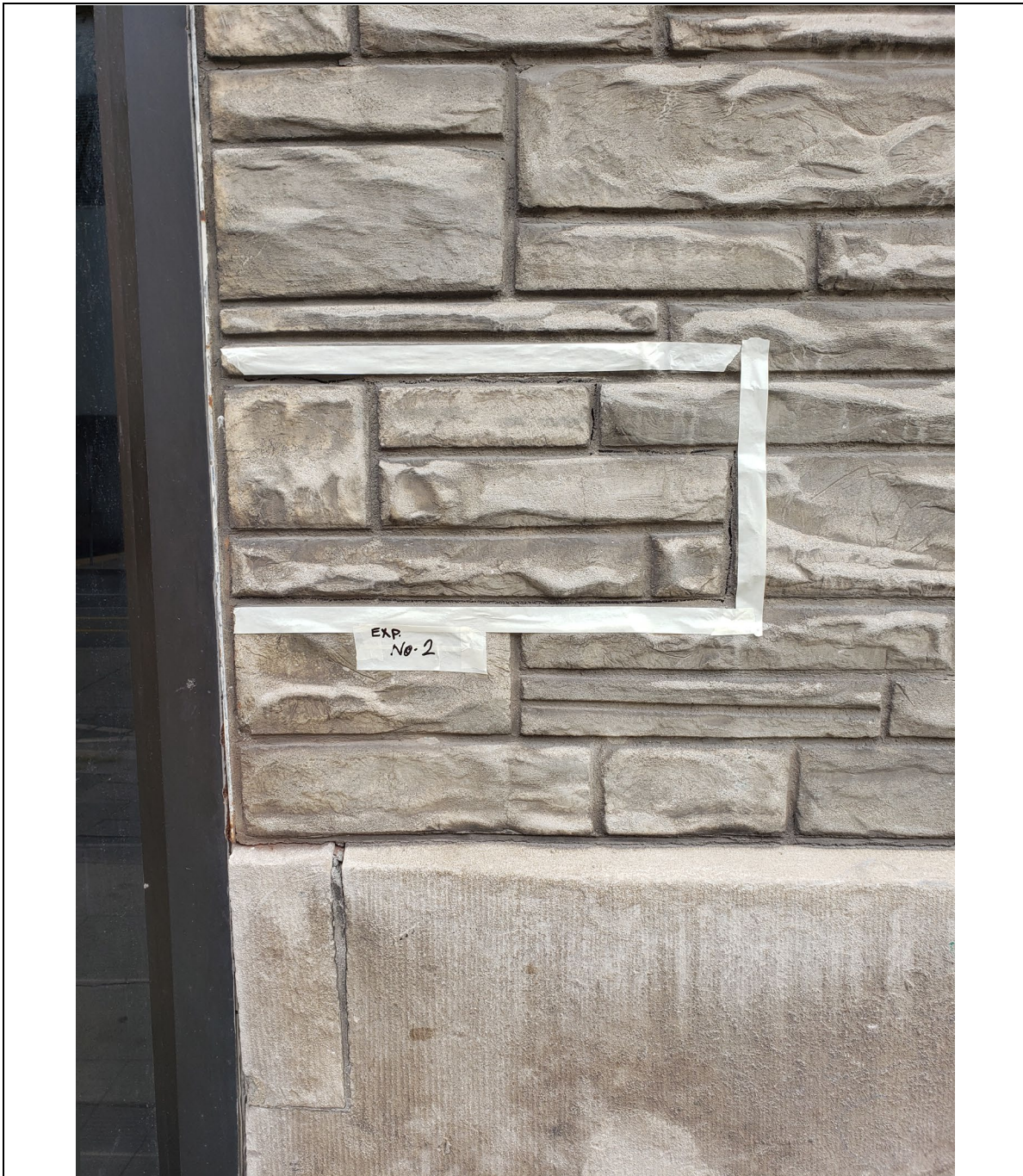
Photograph No. 22, showing a view of the stonework for Exploratory Opening No. 2, adjacent to the door, prior to removal of the stone.
