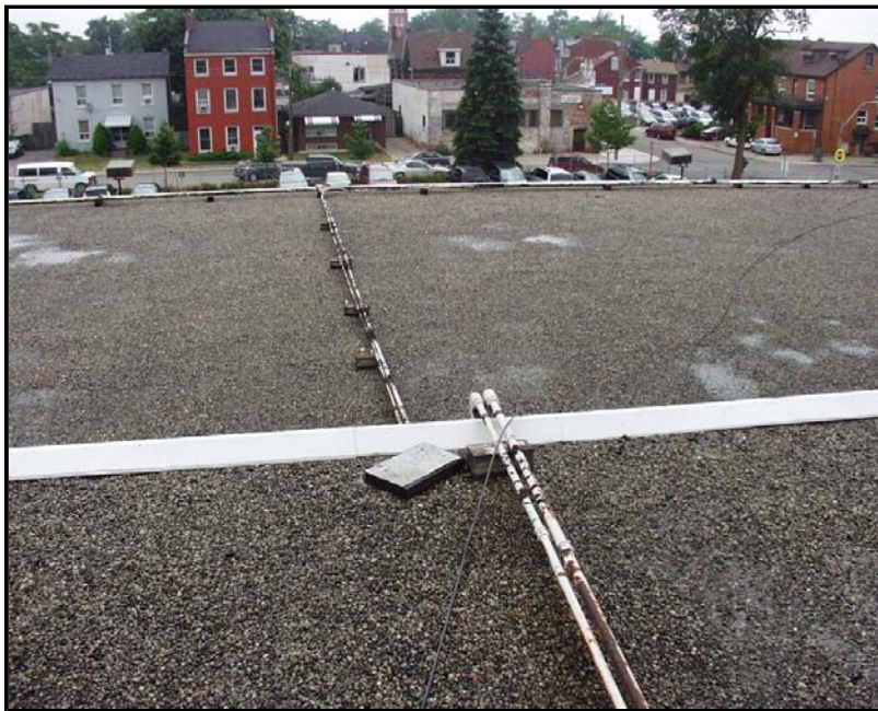
Photo No. 42: Corroded Electrical Conduit
