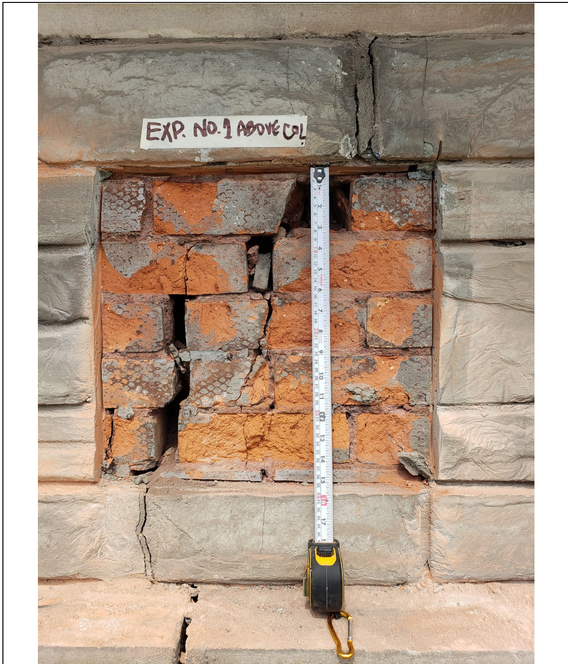
Photograph No. 17, showing a view of the stonework for Exploratory Opening No. 1 after removal of the stone. Note the spalling and cracking seen in the brickwork.
