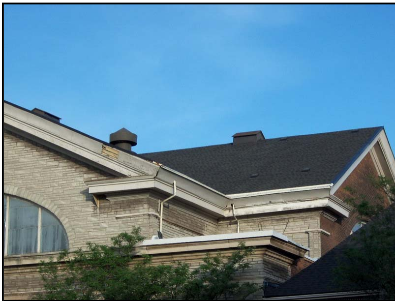
Photo No. 14: Sanctuary sloped roof deteriorated fascia
