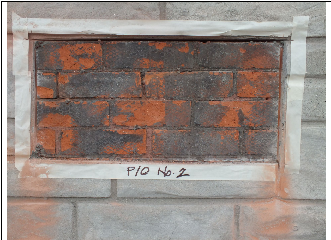
Photograph No. 40, showing the brick work in behind stone facing for Anchor Pull-out Location No. 2. Note the spalled portions of brick.
