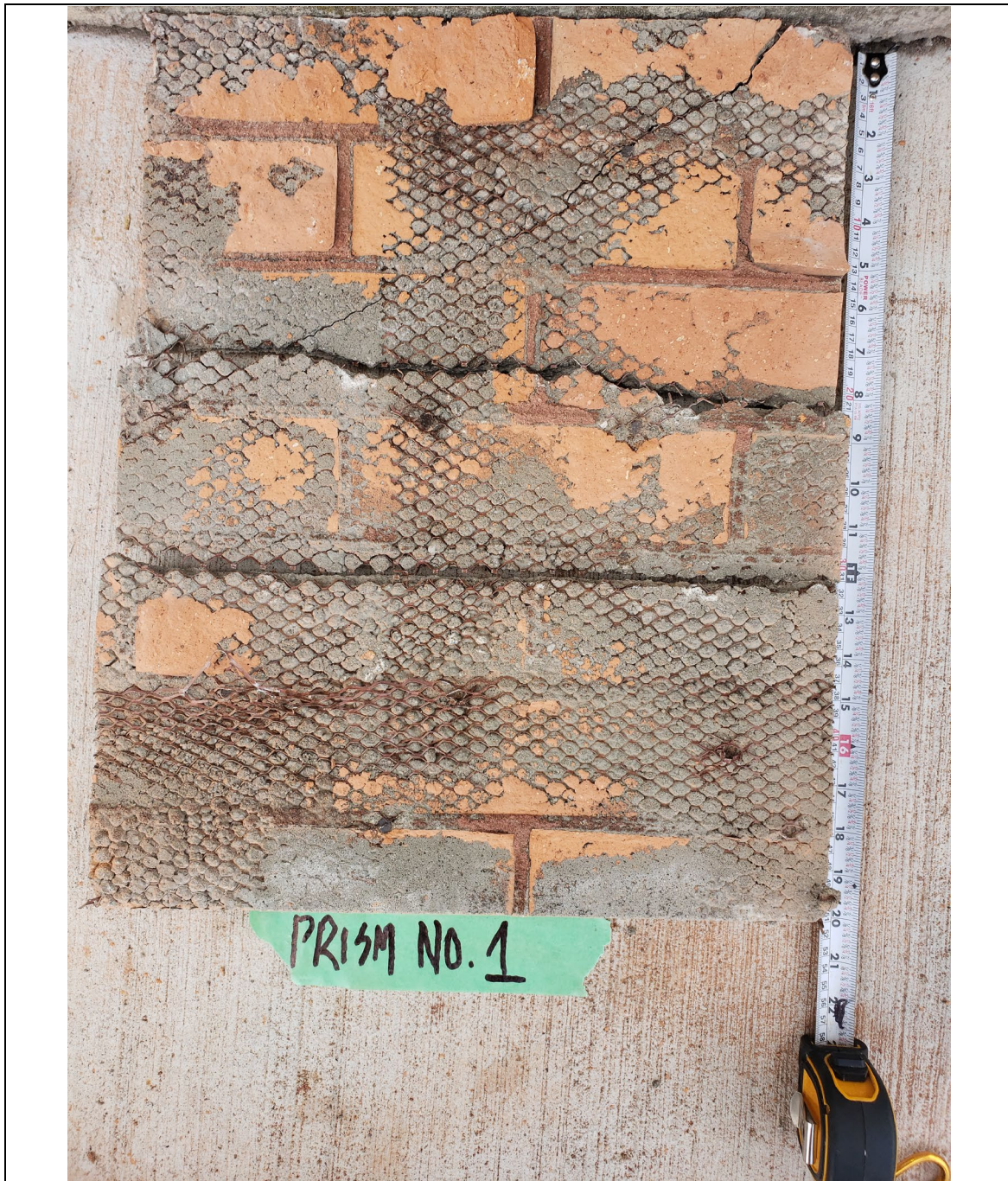
Photograph No. 4, showing test location for Brick Prism No. 1, upon removal of the stone work. Note the visible rusted steel mesh and rusted steel concrete nail heads holding the mesh to the brick. Stonework base mortar was still bonded to the brickwork for most of the area.
