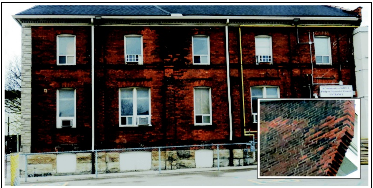
Photo 2 with inset image: There was much evidence of badly-weathered masonry and brick replacement within the side and rear elevations.
