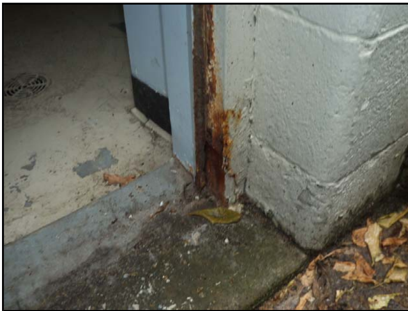
Photo No. 20: Corroded Door Frame at Emergency Basement Exit
