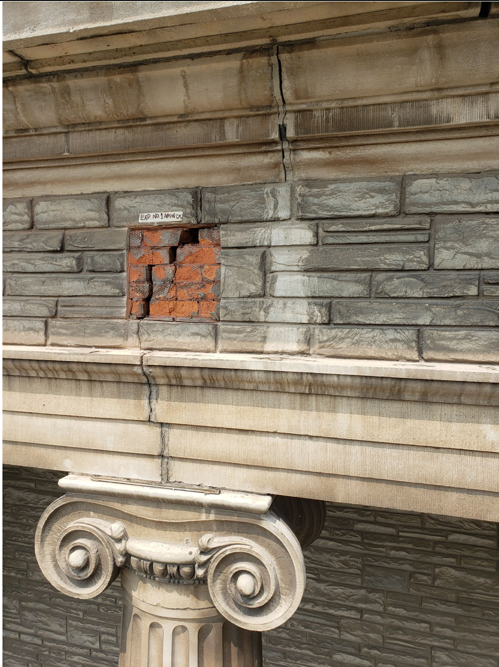
Photograph No. 19, showing an overall view of the stonework for Exploratory Opening No. 1 after removal of the stone. Note the open joints above and below the opening, which likely allows water to penetrate the masonry work and cause freeze-thaw damage to the brick work.
