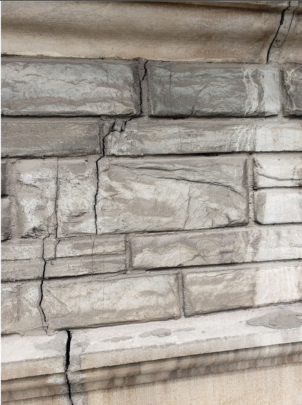
Photograph No. 16, showing a view of the stonework for Exploratory Opening No. 1 prior to removal of the stone. Note the cracking seen in the stonework.
