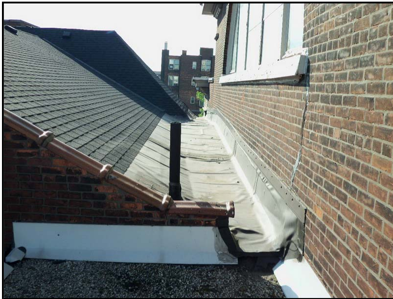
Photo No. 12: Roofing membrane at Original Building
