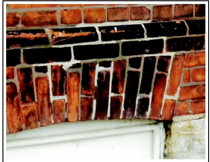
Photo 3: Evidence of several attempts at repointing cracked or deteriorated mortar joints adjacent to window openings
