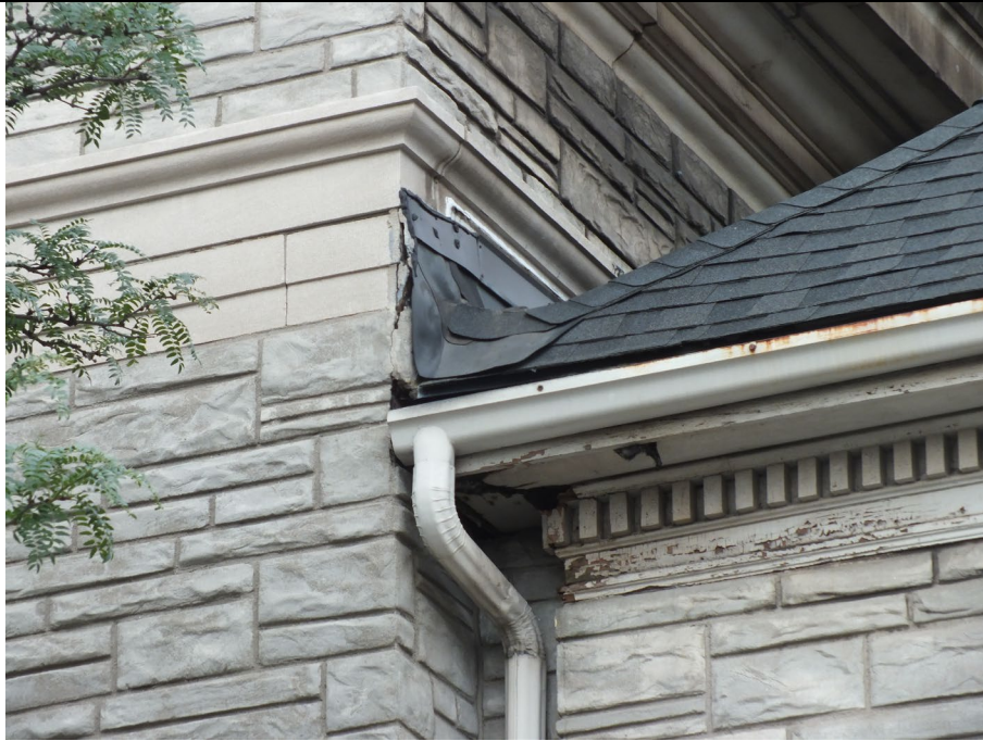
Photograph No. 20, immediately above the eave's trough, separation of the stonework was noted. Note the shingles covering this area.
