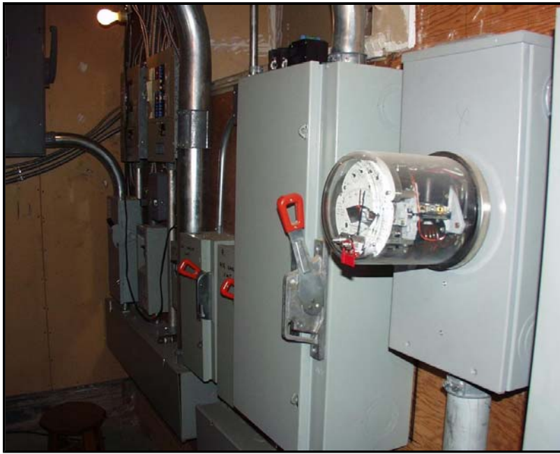
Photo No. 41: Typical Electrical Disconnects
