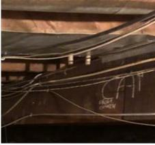
It is recommended that all the full extent of the knob and tube wiring elements be determined and replaced with modern electrical components. Due to the unknown details regarding this item a firm cost estimate for the recommended work cannot be determined, however an estimate is provided that includes a high contingency allowance in order to account for unknowns with this type of work.
