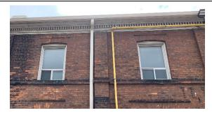
Original window openings with wood sills, lintels and hood molds
