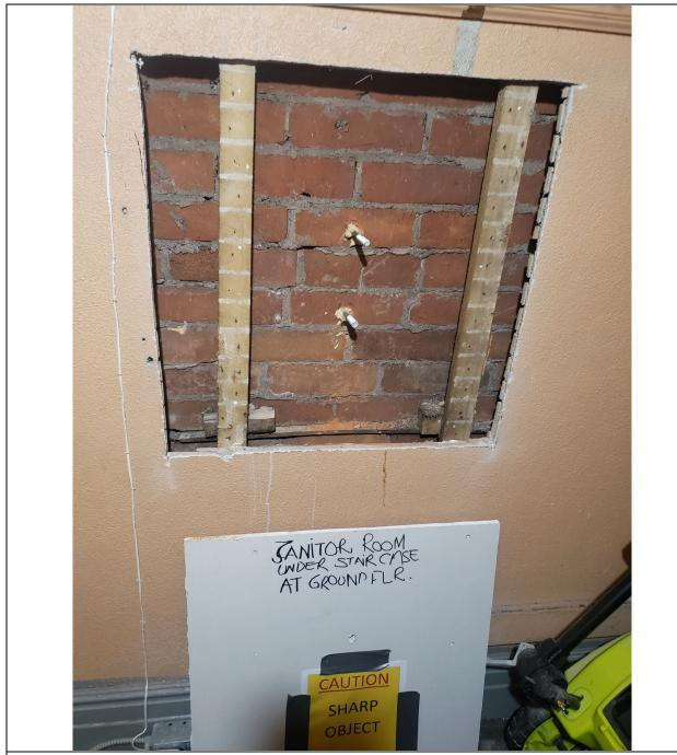
Photograph No. 41, showing anchor bolt installation for Anchor Pull-Out Location No. 4.
