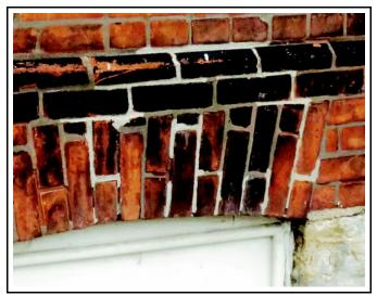
Photo 3: Evidence of several attempts at repointing cracked or in a concentration of gravity loads at the deteriorated mortar joints adjacent to window openings
