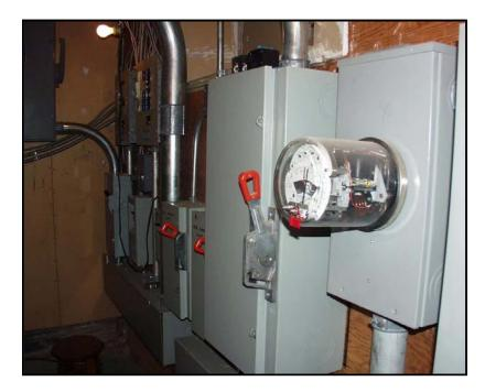
Photo No. 41: Typical Electrical Disconnects
