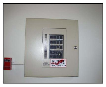
Photo No. 36: Fire Alarm Panel
