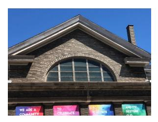
Windows on the 1968 Atrium addition are also of an unconfirmed vintage, but based on observations appear that they may date from the original construction of the Atrium. These windows are set high in the elevations and therefore difficult to assess, however, they do appear to be vertical sliding type windows with metal
