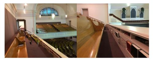
In order to correct this a possible solution is to install a handrail on top of the wall to the minimum heights required by the OBC. This could be a simple upgrade, but at a moderate cost point.
