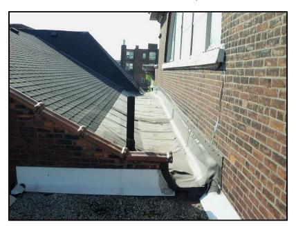
Photo No. 12: Roofing membrane at Original Building
