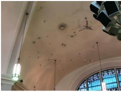
The walls in the Sanctuary, including the balcony fronts, are also suspected to be a plaster material including some decorative detailing. No major issues were noted with the walls, however, if work were to be completed on the ceiling it would be recommended to include completion of any needed minor repair and refinishing work on the walls at the same time
