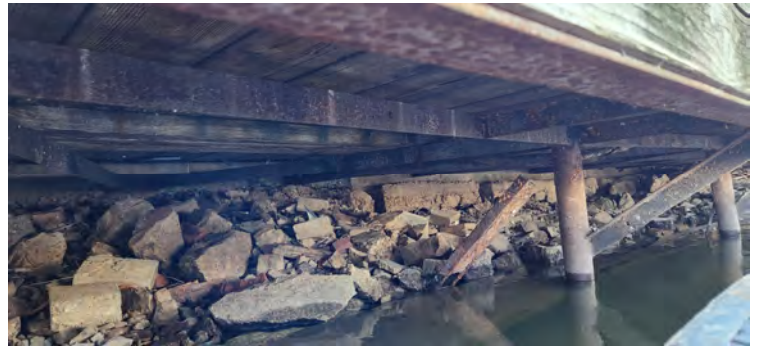
Photo 4: View Below the Deck Which Show the Exposed Foundation
