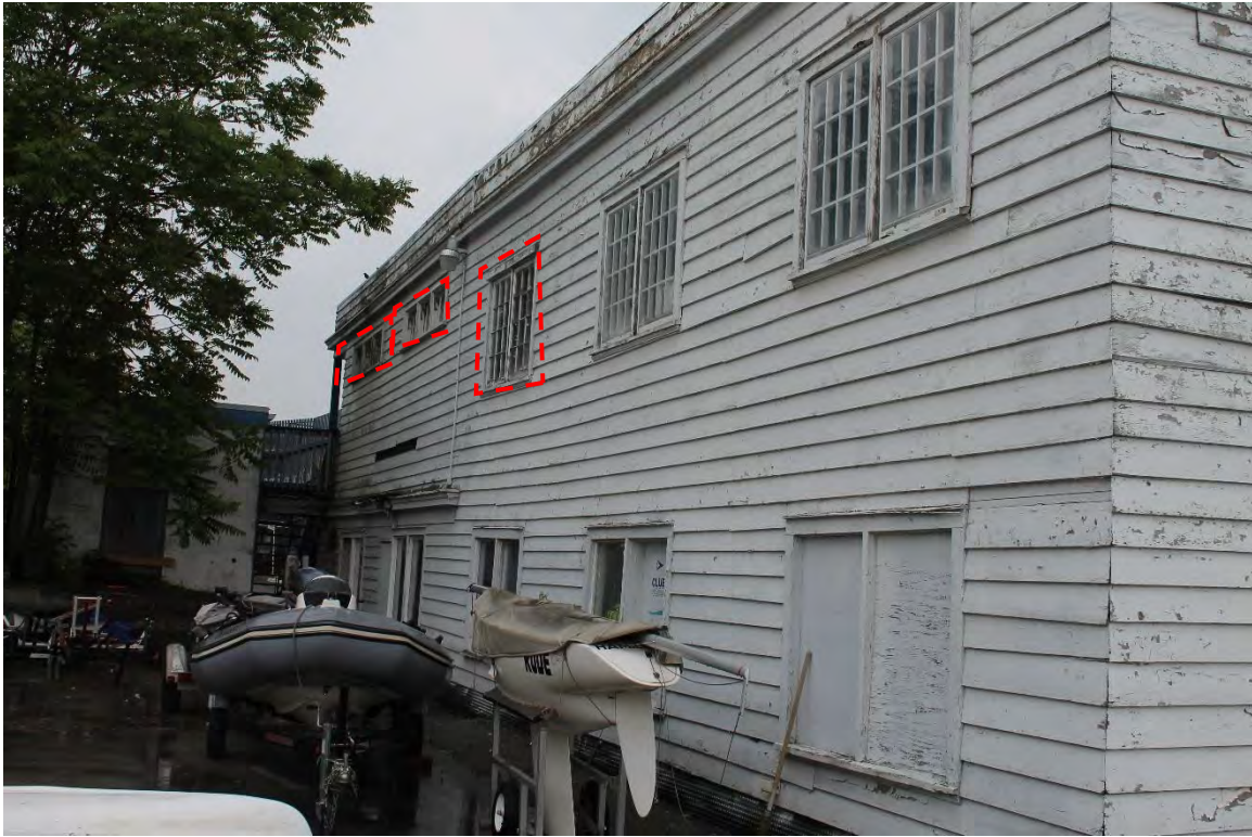
Figure 19: View of south façade of the Sailing School Facility noting the location of mid. 19 th century wood windows which may be candidates for salvage provided that they are in good condition (Source: MHBC, 2023).
