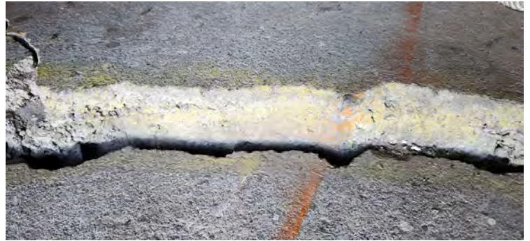
Photo 3: Close Up View of the Cracked Slab Inside the Lockers
