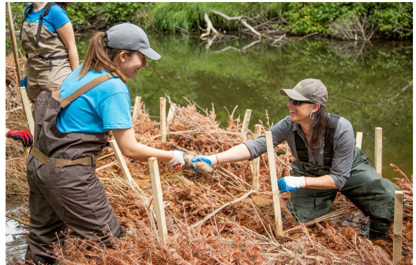
Restoration team using donated Christmas trees to build river banks
