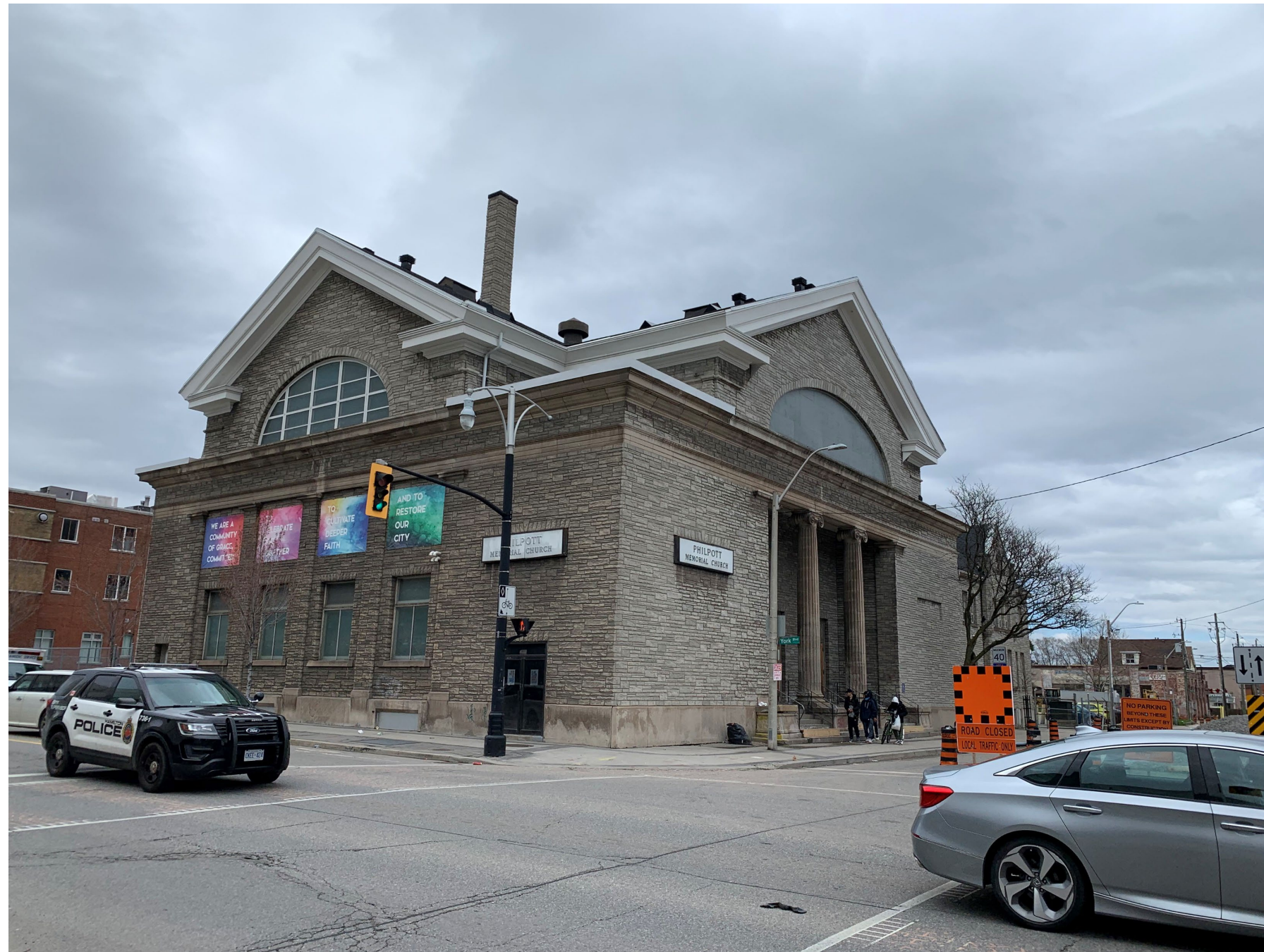
1906 façades covered with cement-based mortar
