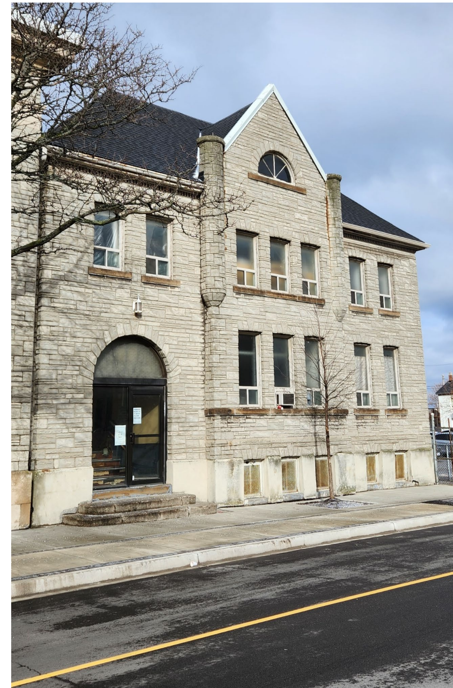
1901 façade covered with cement-based mortar
