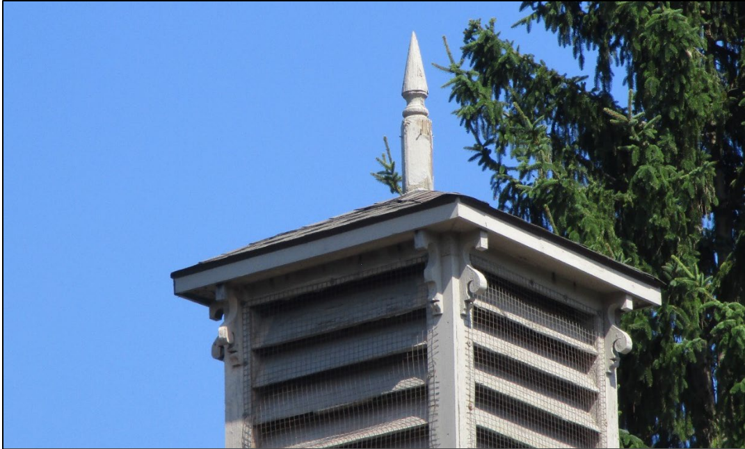
Image 19: Detail of Finial on Cupola on Coach House
