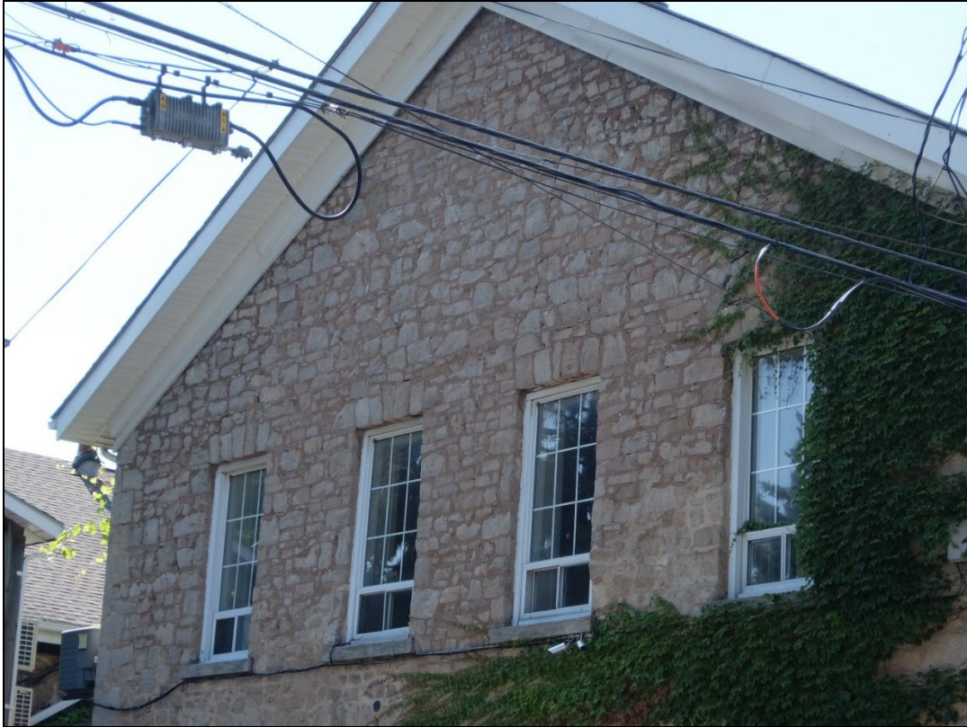
Image 8: Masonry Detail of Second Floor of Rear (East) Elevation of Hotel
