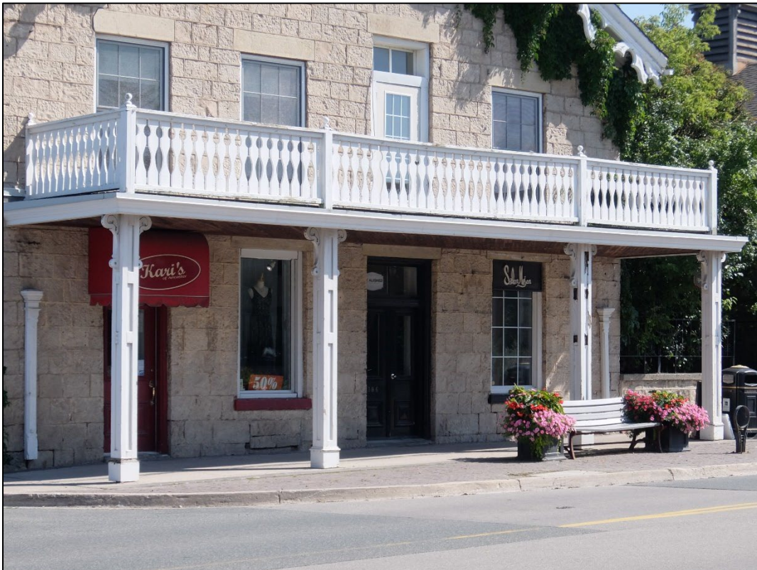
Image 11: Detail of Main Floor on Front (West) Elevation of Hotel
