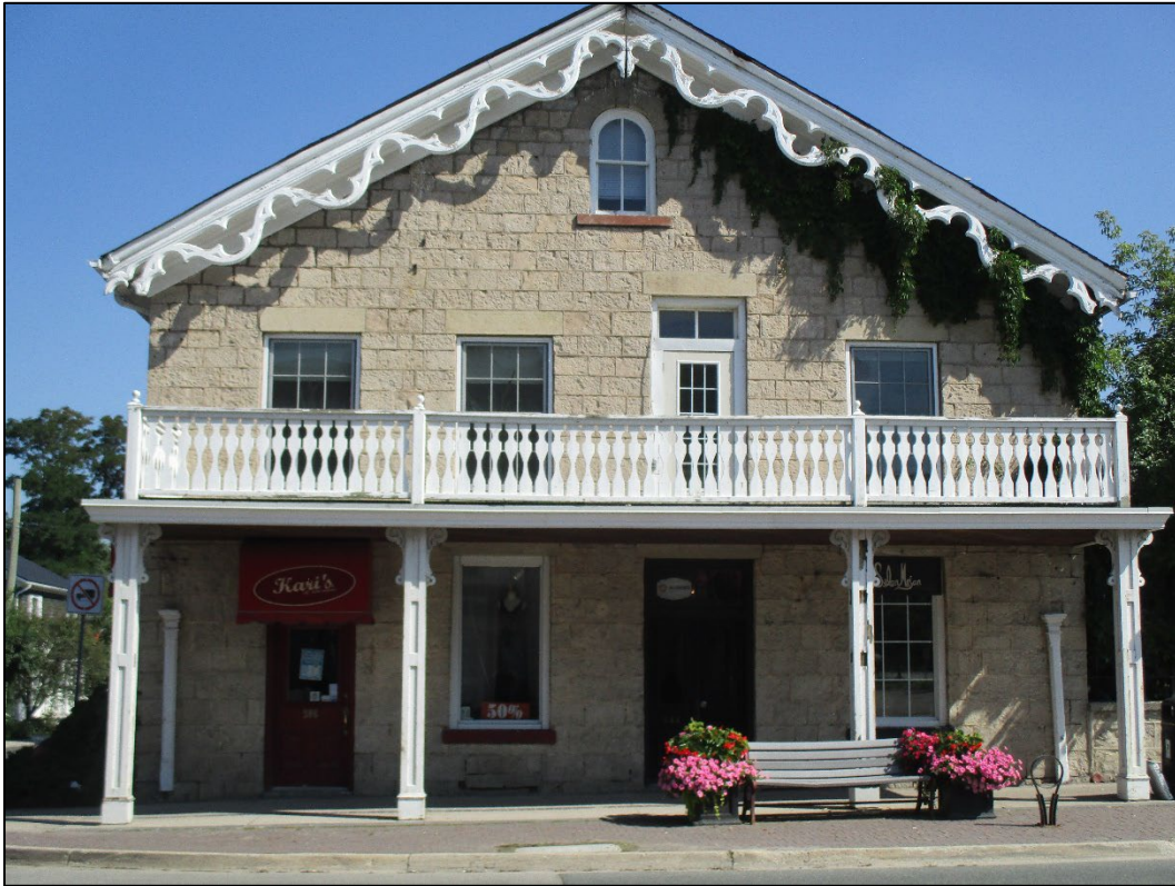
Image 3: Front (West) Elevation of Hotel
