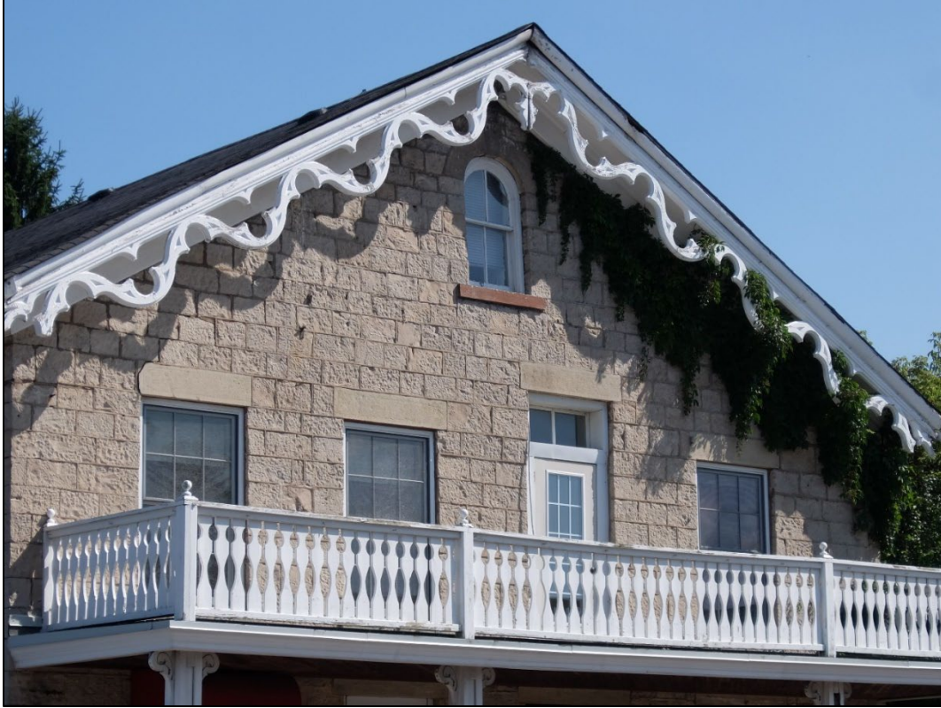
Image 10: Detail of Second Floor on Front (West) Elevation of Hotel
