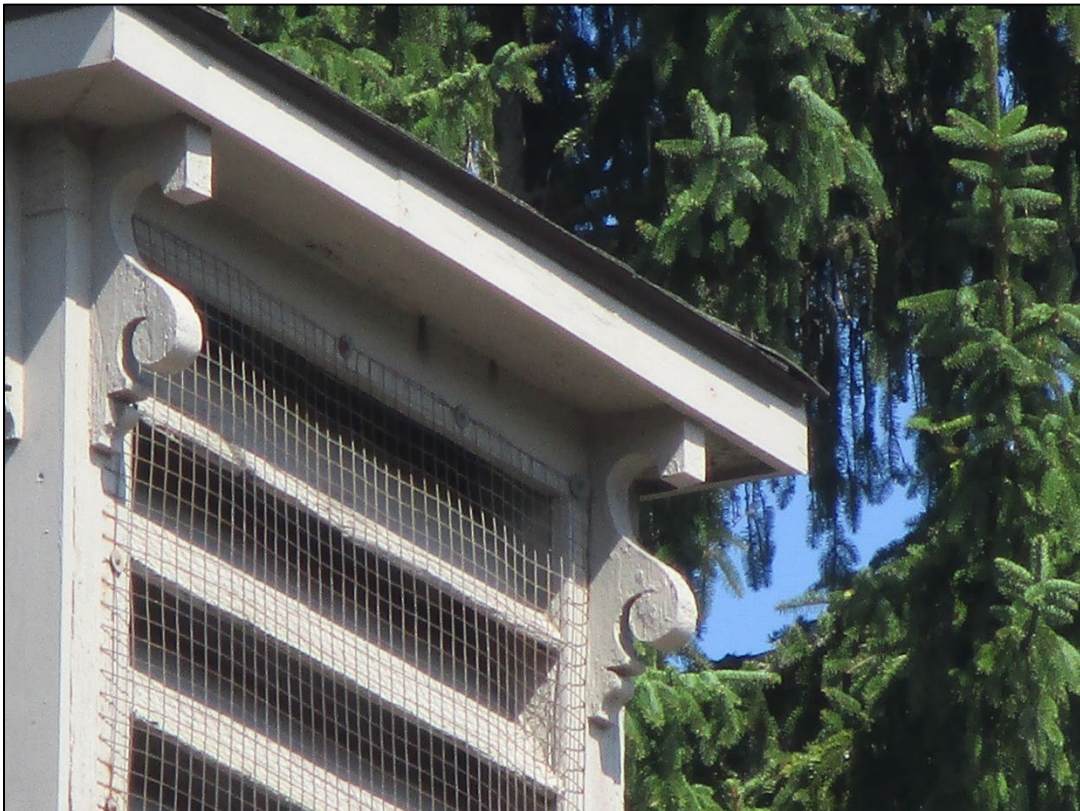
Image 20: Detail of Brackets on Cupola of Coach House
