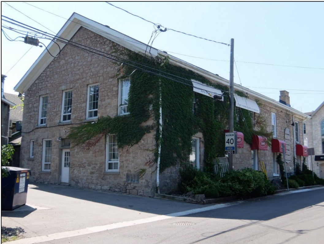
Image 6: Side (East) and Rear (North) Elevations of Hotel
