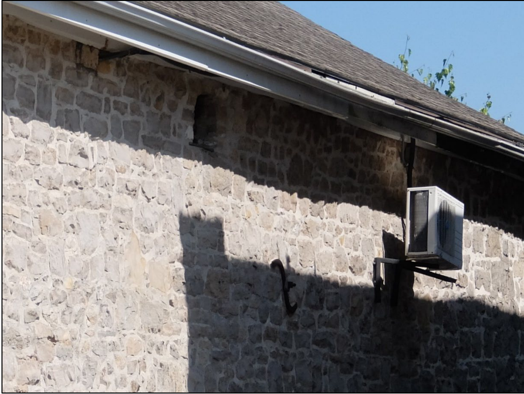
Image 17: Masonry Detail on Side (South) Elevation of Coach House
