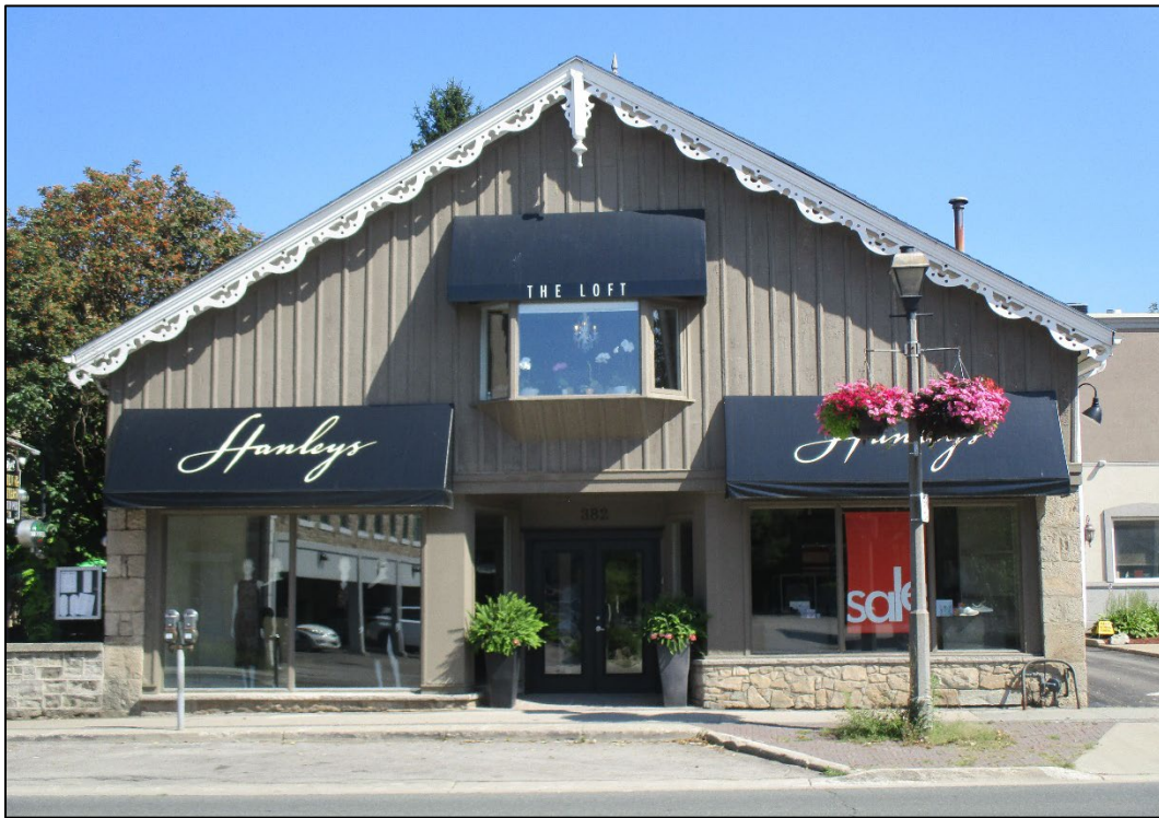
Image 4: Front (West) Elevation of Coach House
