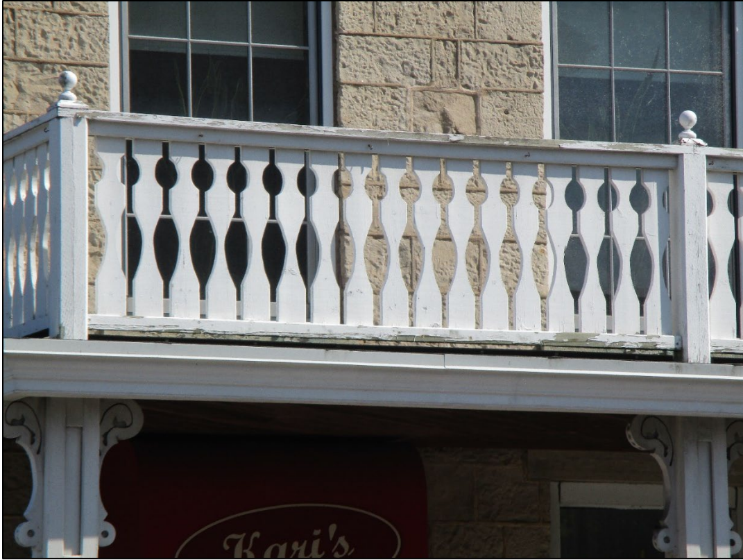
Image 13: Detail of Balcony Railing on Front (West) Elevation of Hotel
