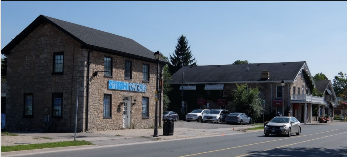
Image 22: Streetscape view of Subject Property looking South past Academy Street
