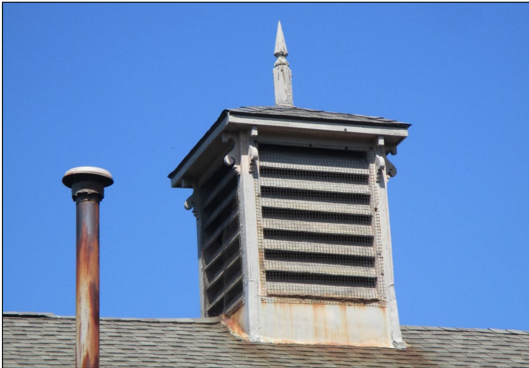
Image 18: Detail of Ventilation Cupola on Coach House
