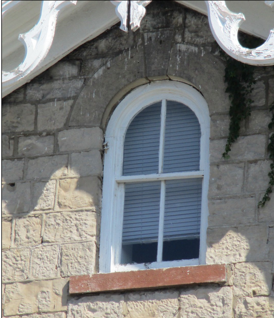
Image 12: Detail of Rounded Wood Window with stone lintel, keystone and sill in the Front (West) Gable of Hotel
