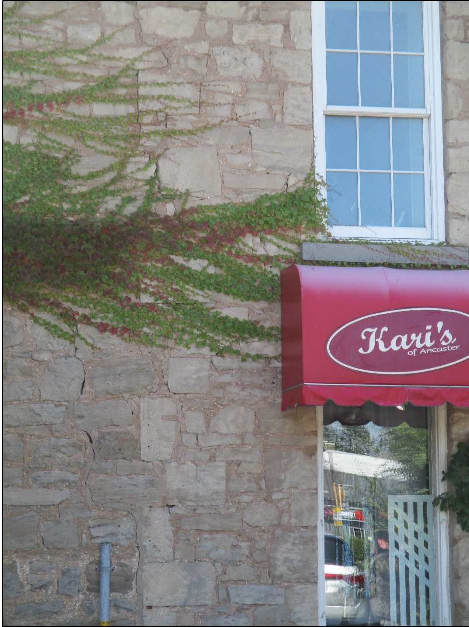
Image 21: Masonry seam detail on Side (North) Elevation of Hotel
