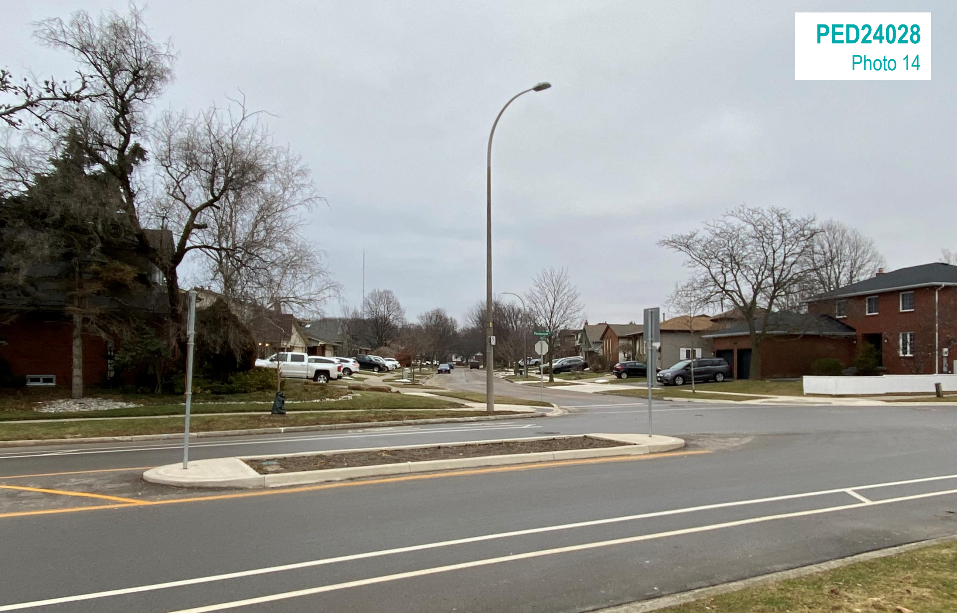
Looking east towards Ackland Street
