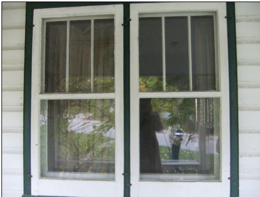
Figure 18: Early twentieth-century windows on front exterior
