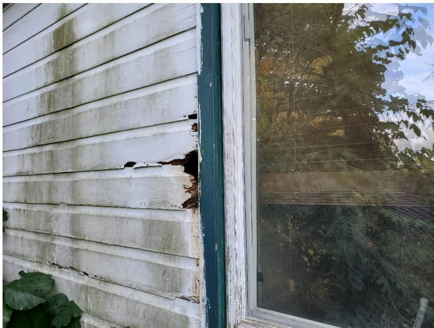
Photo No 06: Rotted Siding
