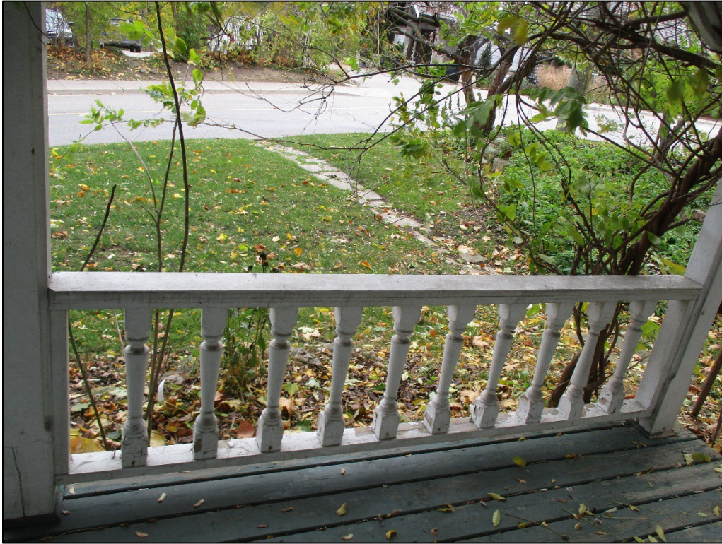
Figure 21: View of turned railings on front porch
