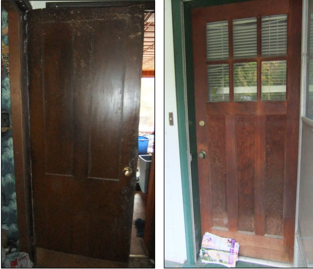
Figure 17: View of interior (left) and front exterior (right) wood doors
