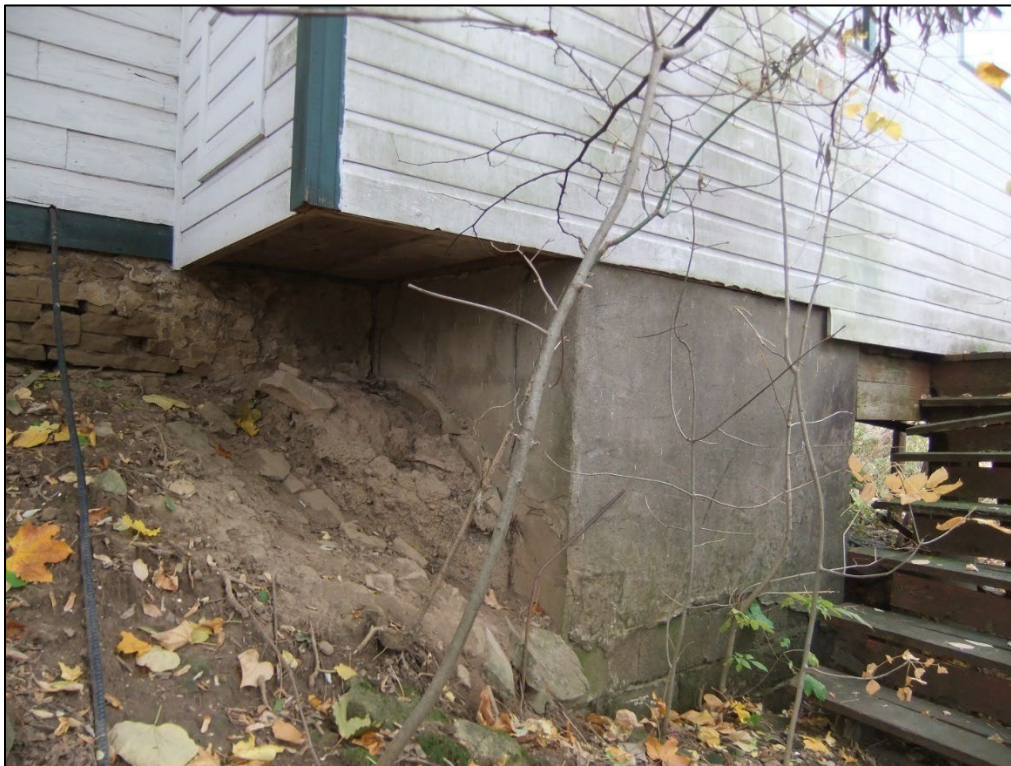
Figure 12: View of contemporary side addition and foundation
