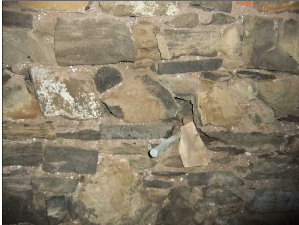
Figure 14: View of stone foundation wall in basement
