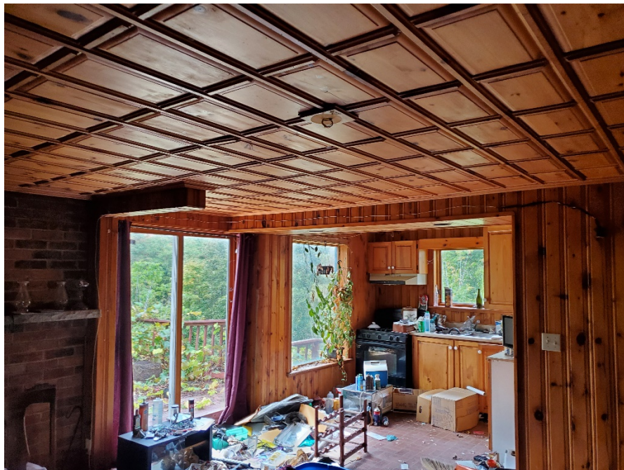
Photo No 02: North Kitchen Wall below Photo No:01
