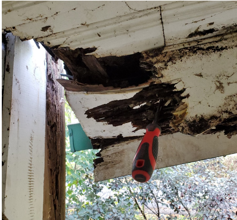
Photo No 05: Rotten Wood
