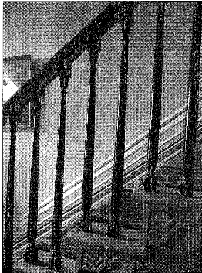
Figure 42: Detail of staircase
