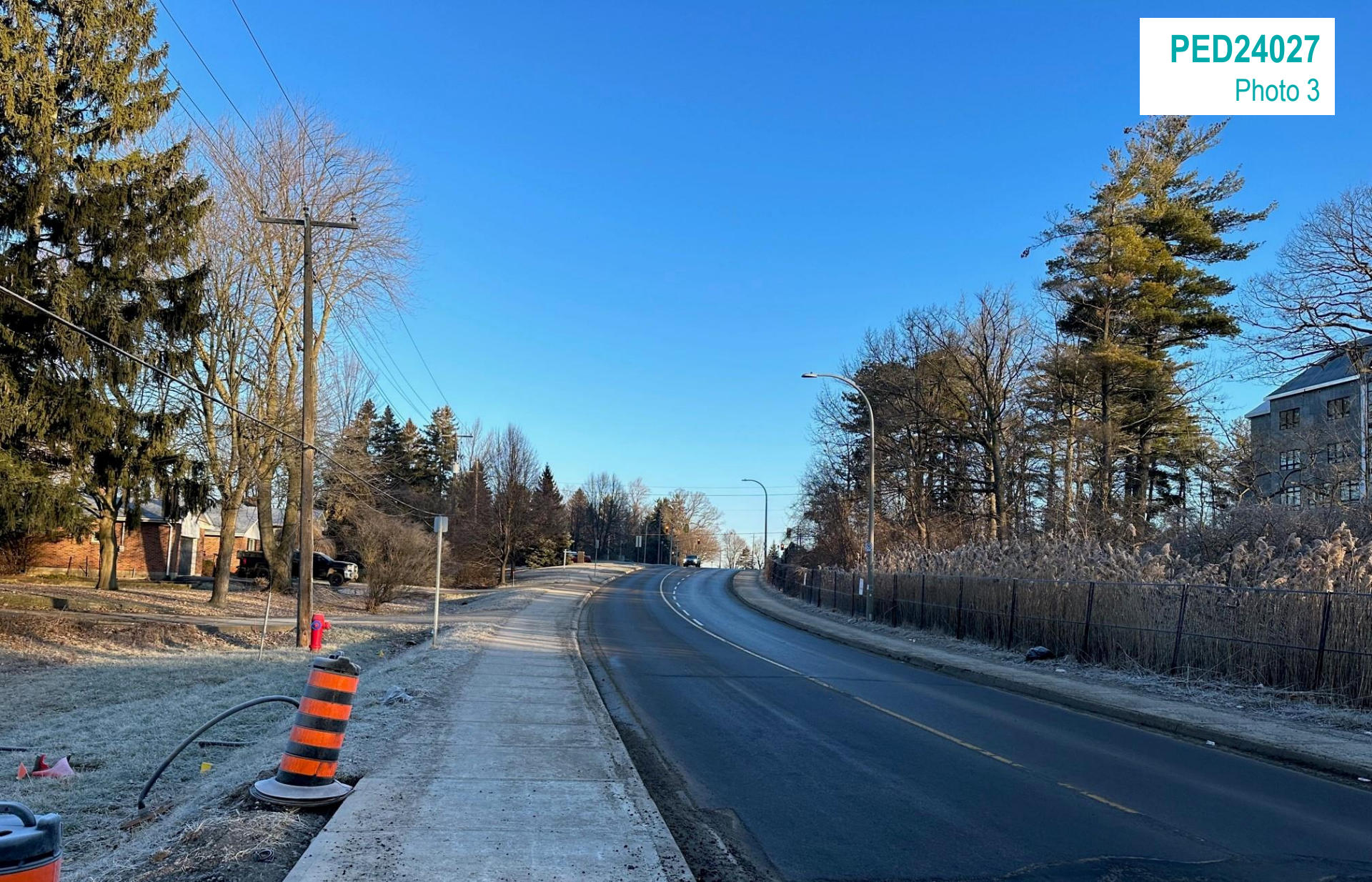
26 Southcote Road - Facing North
