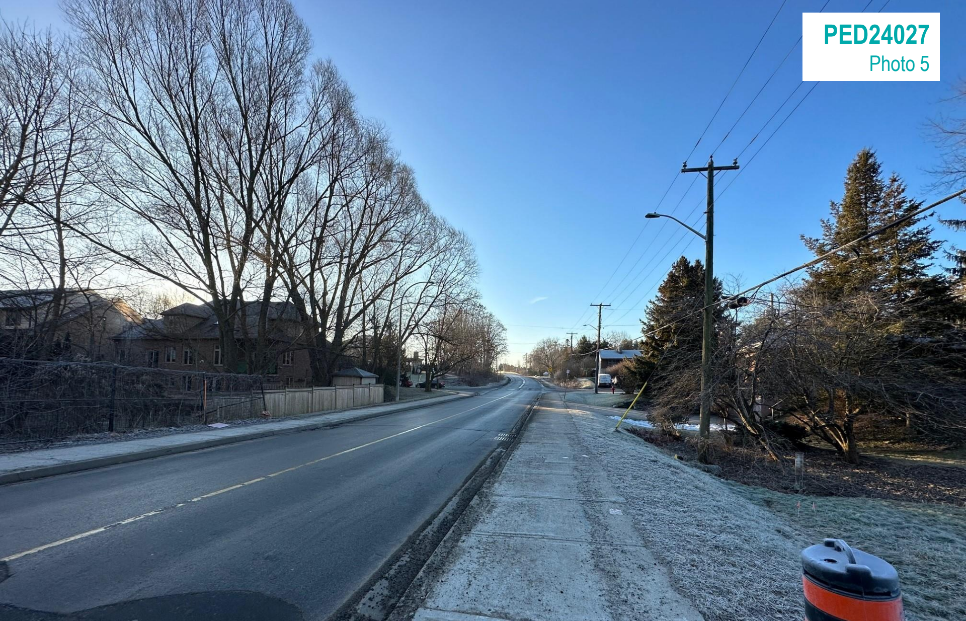
26 Southcote Road - Facing South
