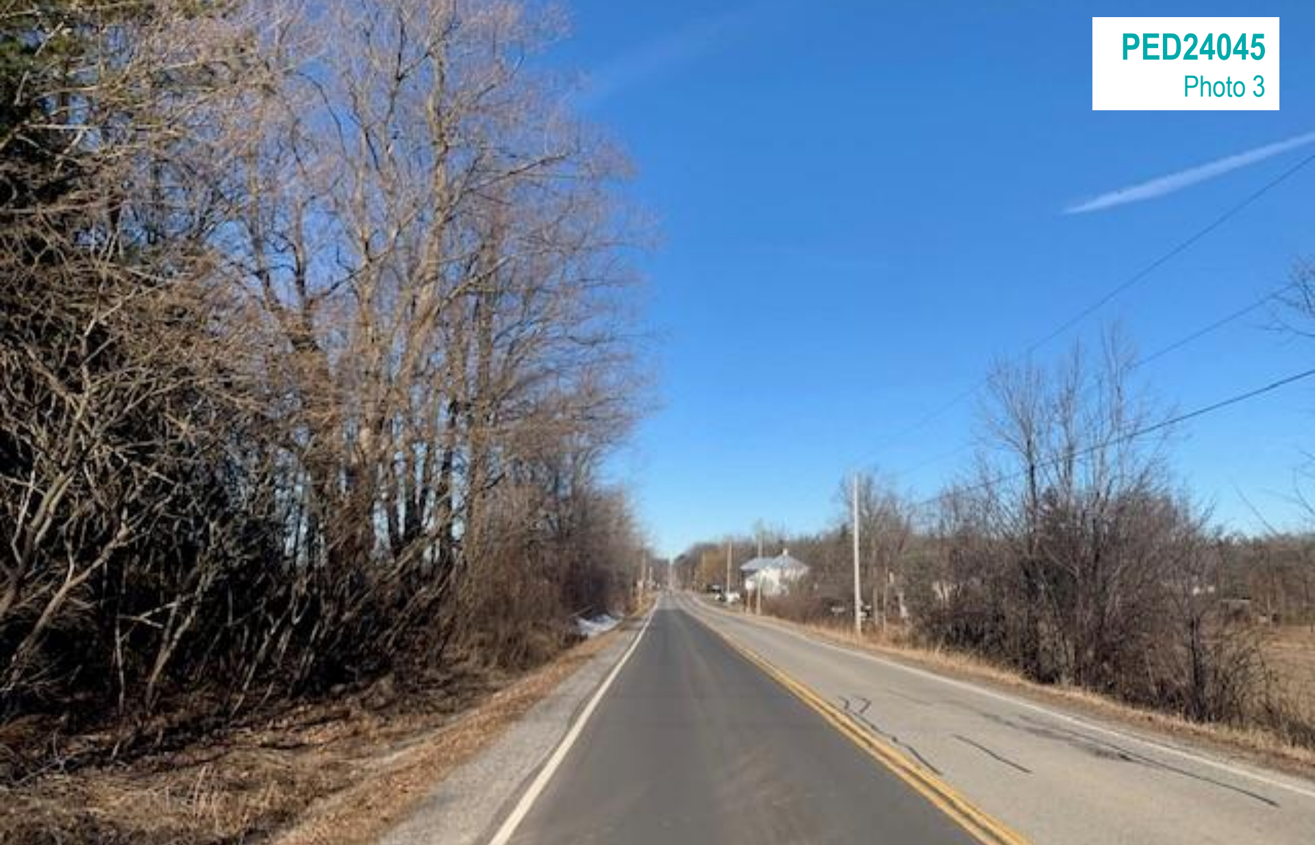
Looking North along Centre Road
