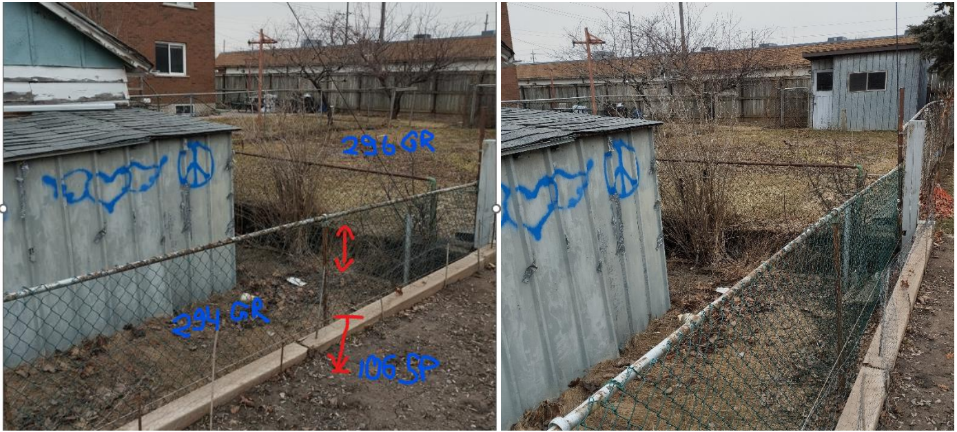
Fig. 3. Images highlighting lower grade of 294 Green Road with retaining walls separating it from 296 Green Road and 106 Seaton Place Drive (red arrows).
