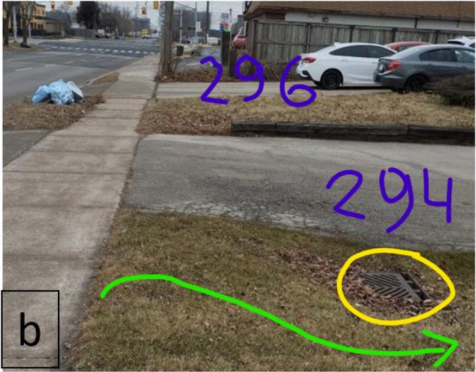
Fig. 4. (a) Location of retaining wall (red line) and catch basins (blue and yellow X). (b) Downward slope of 294 Green Road with the catch basin (yellow) near the high point compared to even grade of 296 Green Road.
