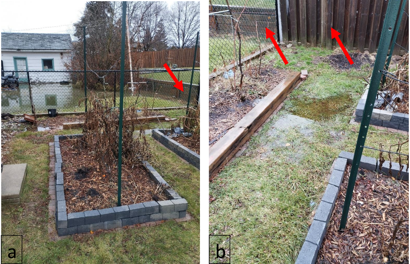
Fig. 2. Flooding of 294 (a) and 292 Green Road (b) during fall 2023 with retaining wall between 106 Seaton Place Drive.
