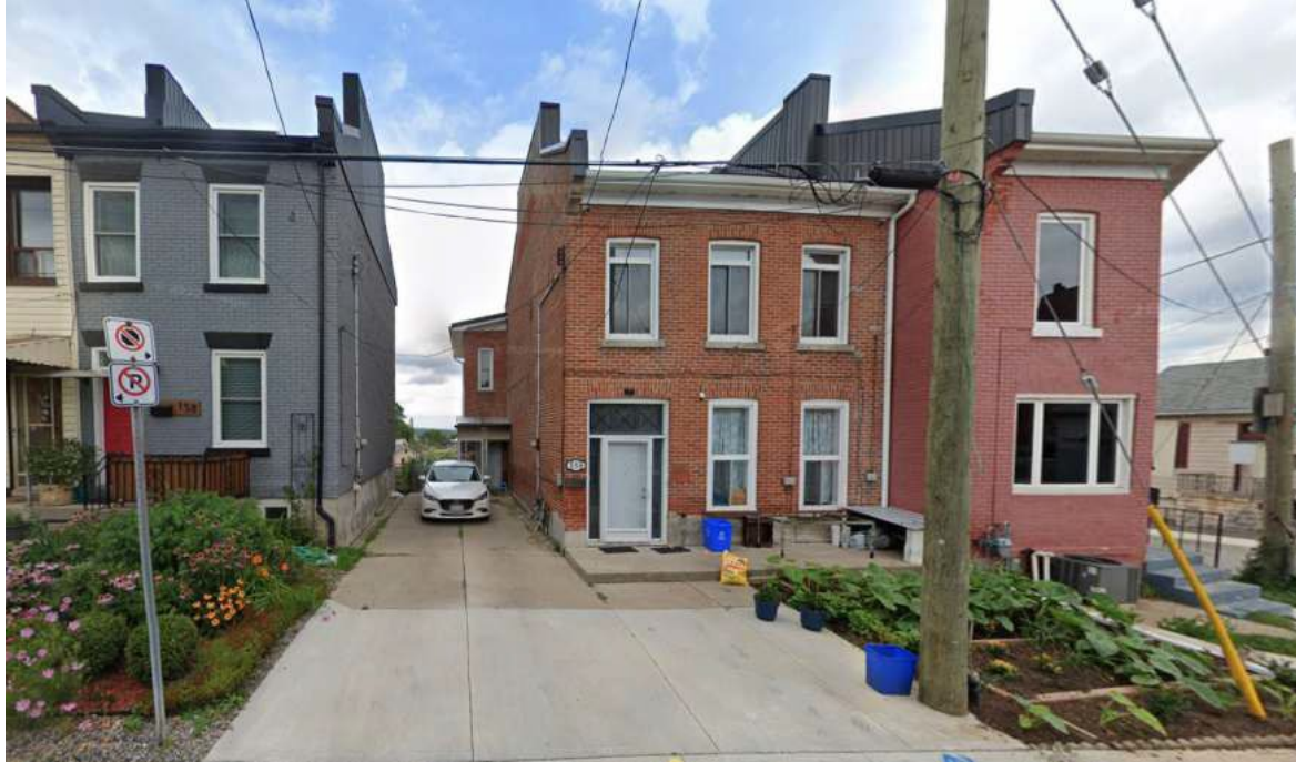
(Fig. 6 Neighbouring front yards along Cannon Street West to the East of the subject property.)
