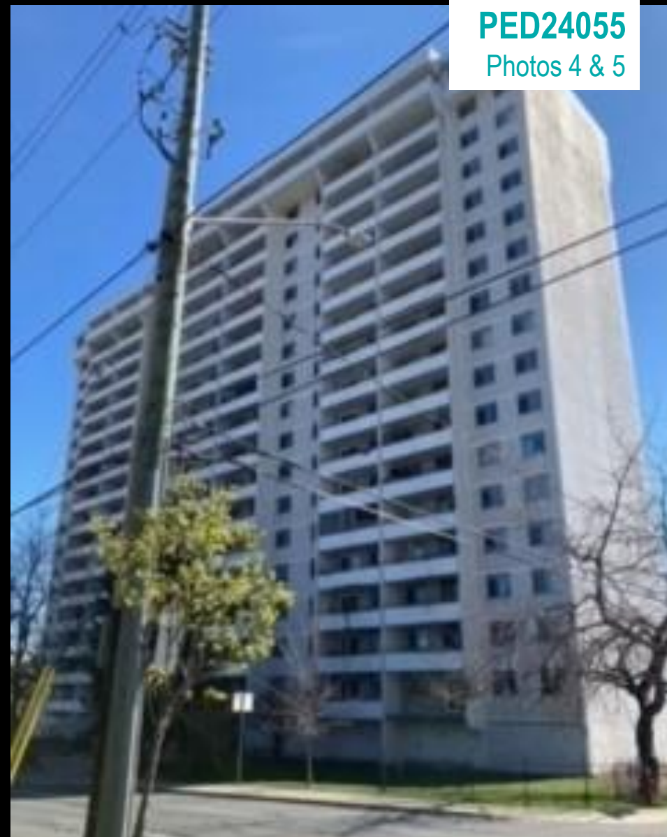
View From the Site Looking at the West Side of Queen Street South 2
