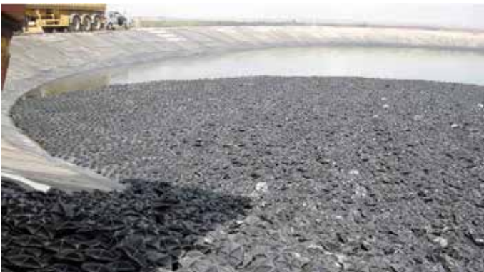
Hexa-Cover ® BULK delivery and installation:
