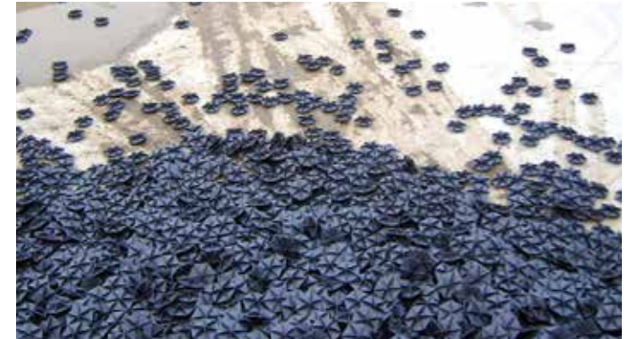
Hexa-Cover ® Also installation in empty tank (max 5m drop)
