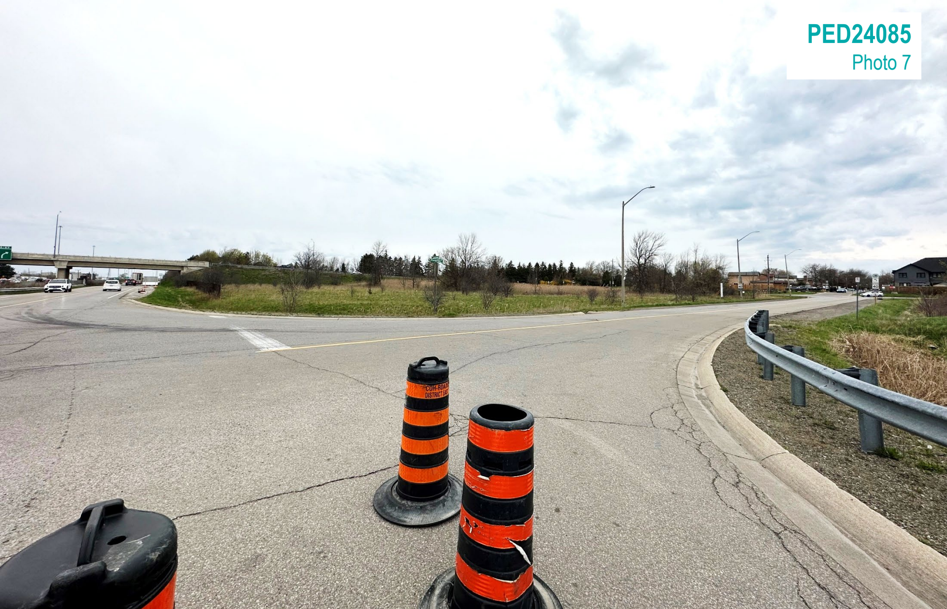
560 Grays Road, SC - Facing Northwest (from Parkedge Drive and Nort Service Road)
