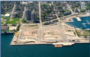
Pier 8 Servicing Infrastructure
