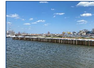
Pier 6&7 Shorewall & Public Boardwalk
