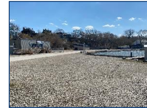
HPS Marine Unit & Rehabilitation
