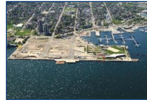
Shorewall Infrastructure Renewal
