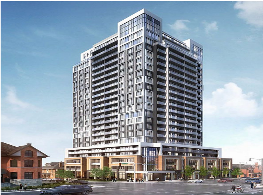
235 Main Street West, Hamilton -Post Construction Rendering (Source: www.apexhamilton.com )
