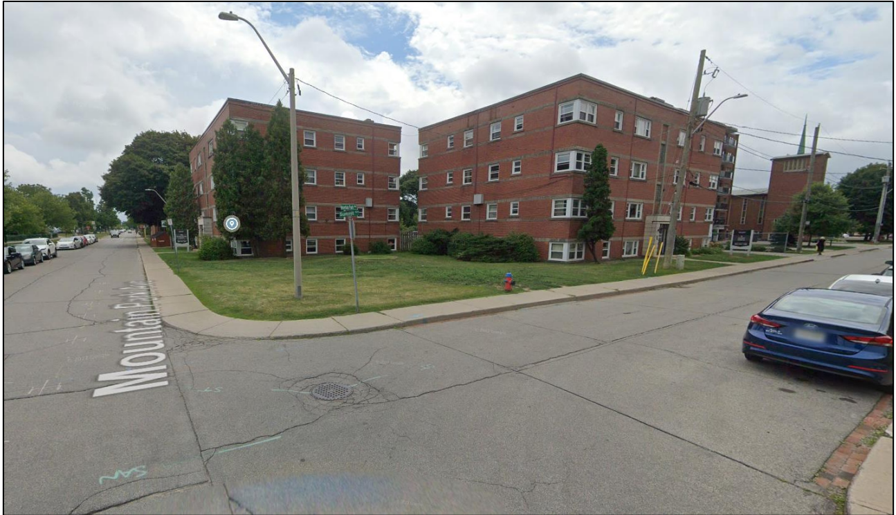
Corner of Mountain Park Ave and Summit Ave
