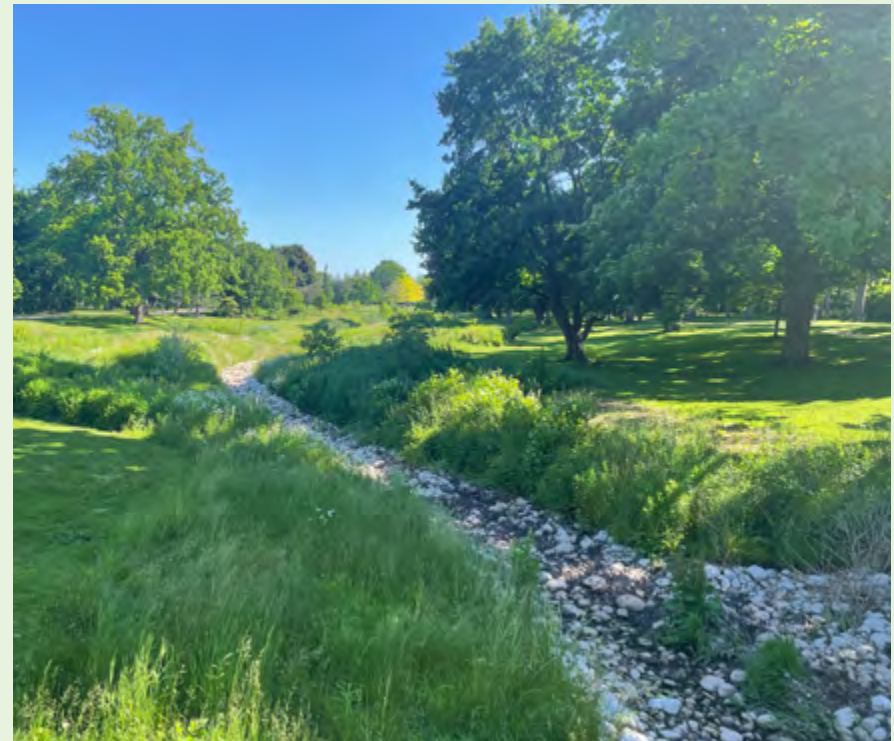
Bioswale in Gage Park. PHOTO City of Hamilton
