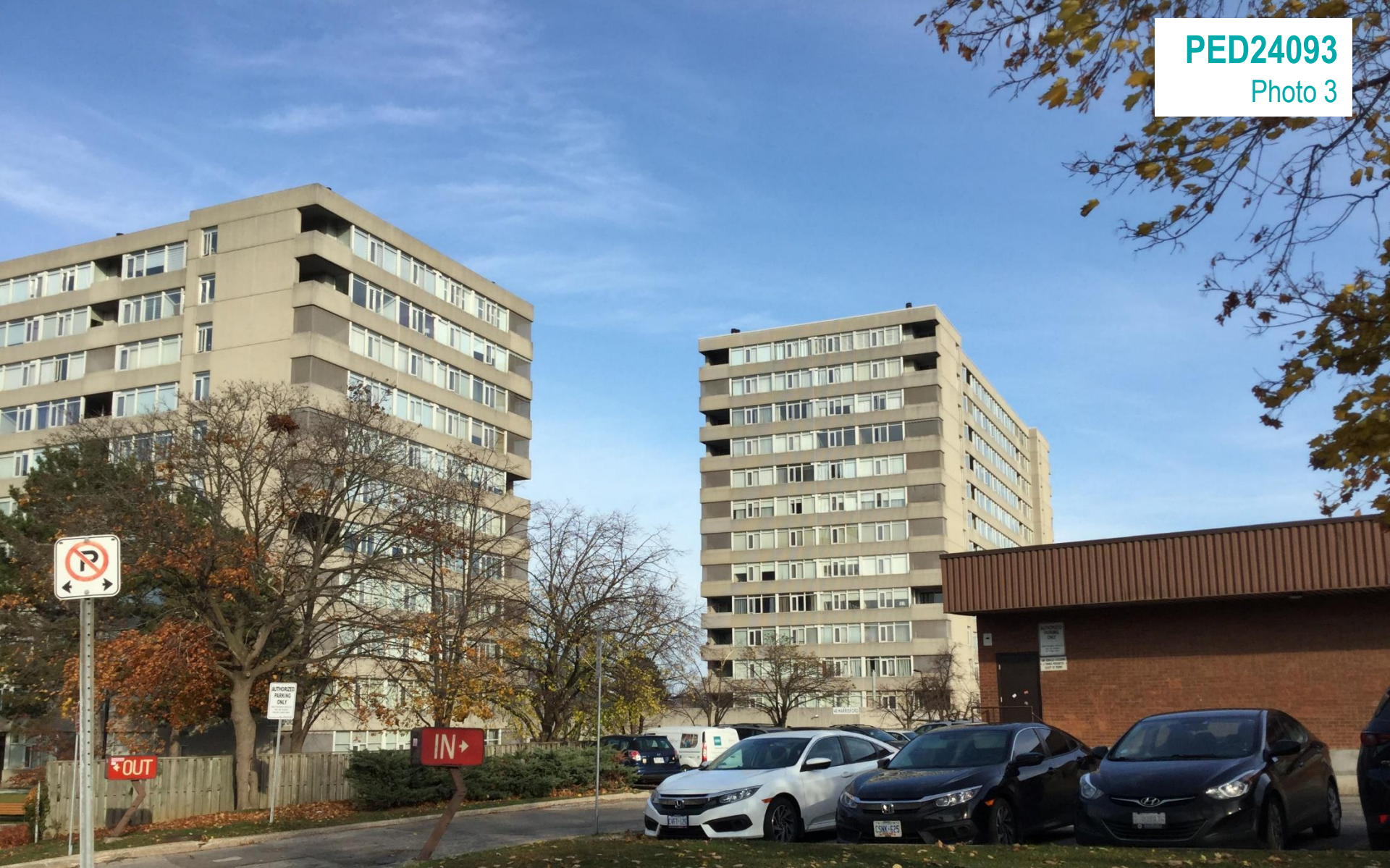
Subject property and the existing 12 storeys multiple dwelling at 30 and 40 Harrisford Street located to the north of the subject property, as seen from Harrisford Street looking north east
