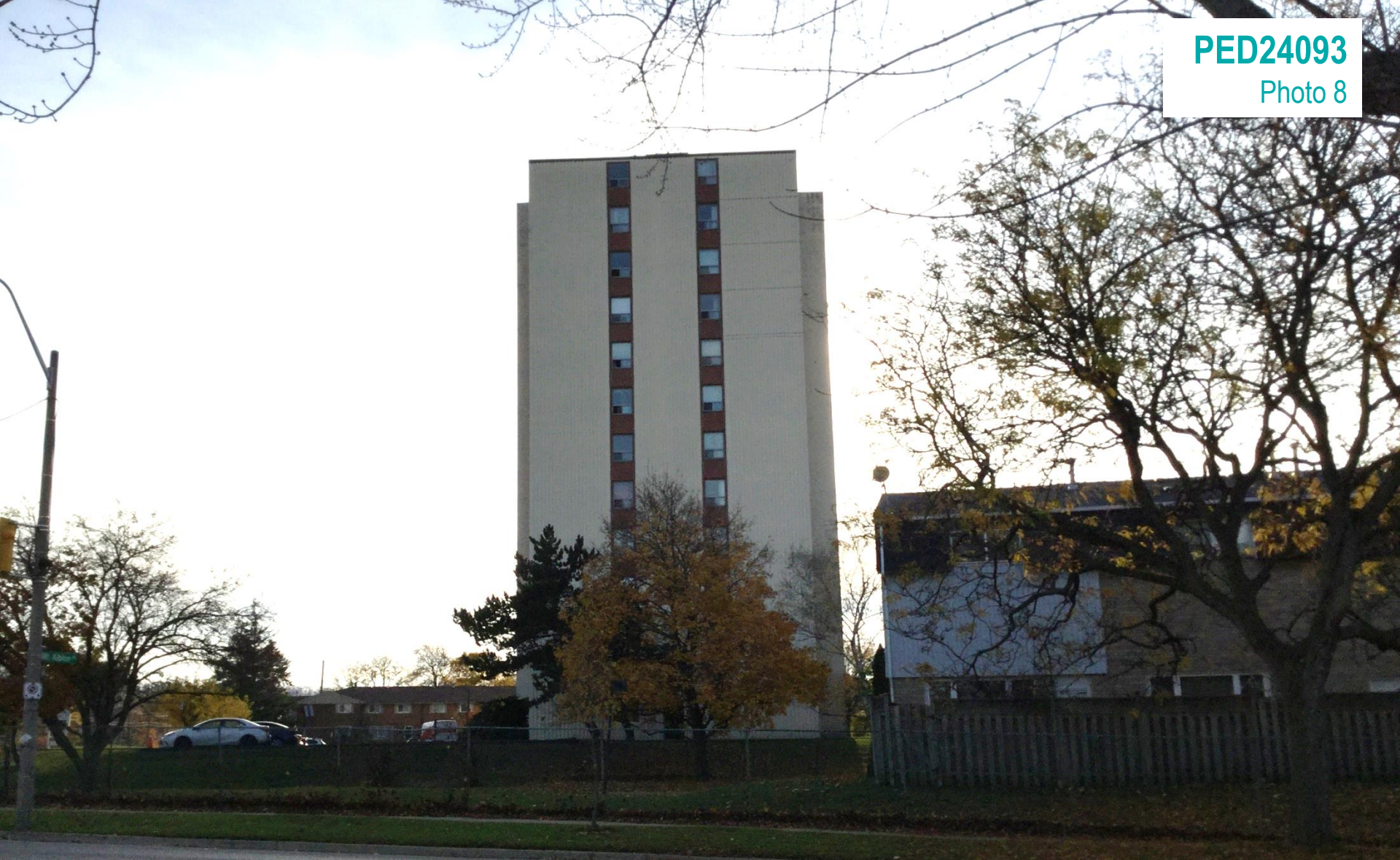
Existing townhouse dwelling and 12 storey multiple dwelling at 288 Mount Albion Road located to the south of the subject property, as seen from Greenhill Avenue looking south
