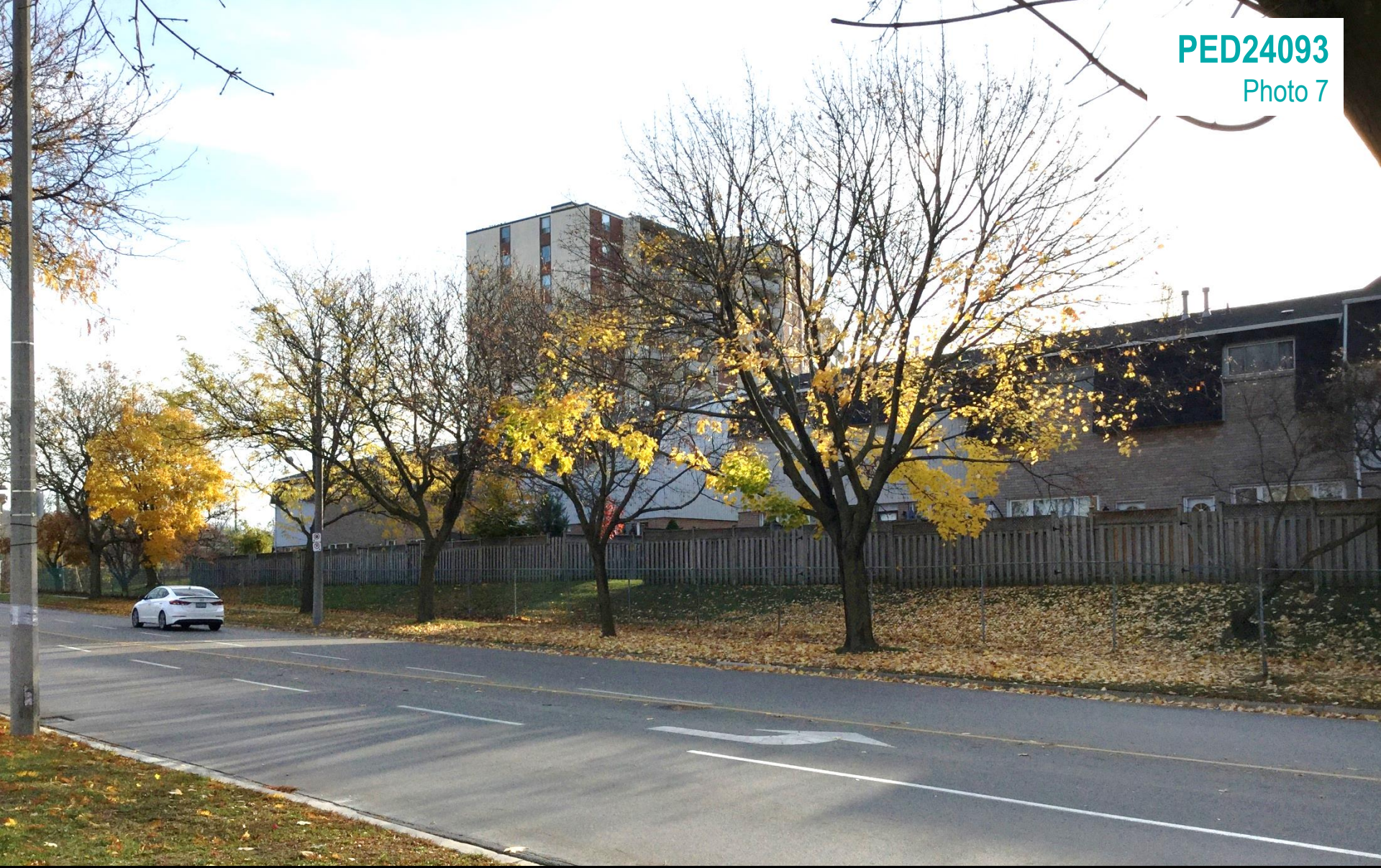
Existing townhouse dwellings and 12 storey multiple dwelling at 288 Mount Albion Road located to the south of the subject property, as seen from Greenhill Avenue looking south east
