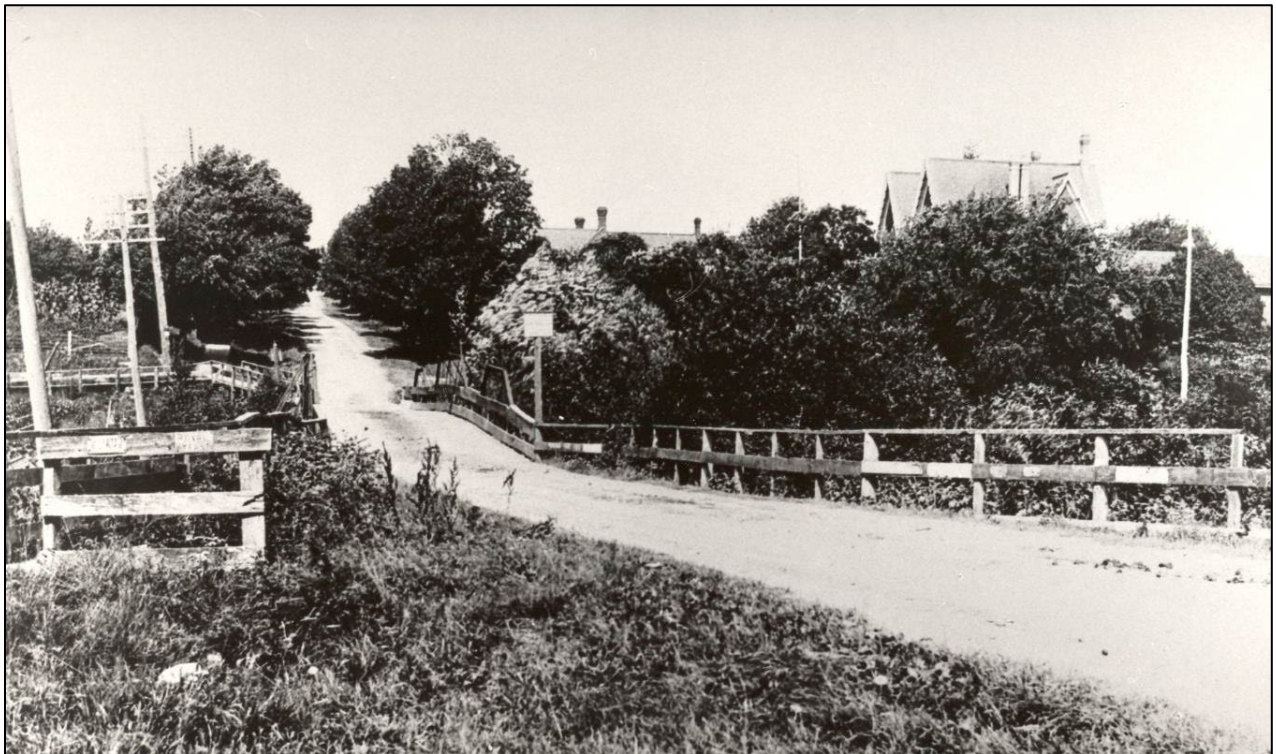
Figure 14: Looking East across Grindstone Creek and up Vinegar Hill. Subject Property on right. c. 1900 (Flamborough Archives)
