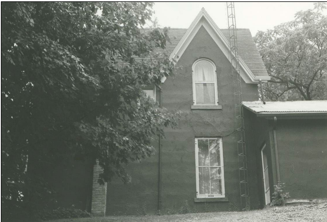
Figure 6: Side (west) elevation, 1982 (Flamborough Archives)
