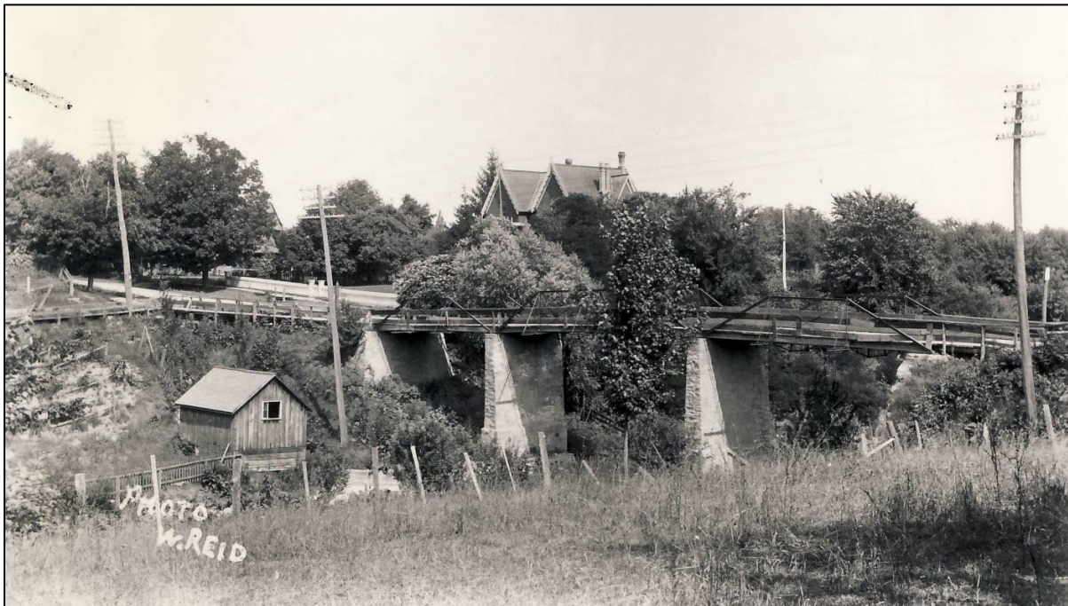
Figure 12: Looking Southeast across Grindstone Creek, c. 1906-1910 (Flamborough Archives)
