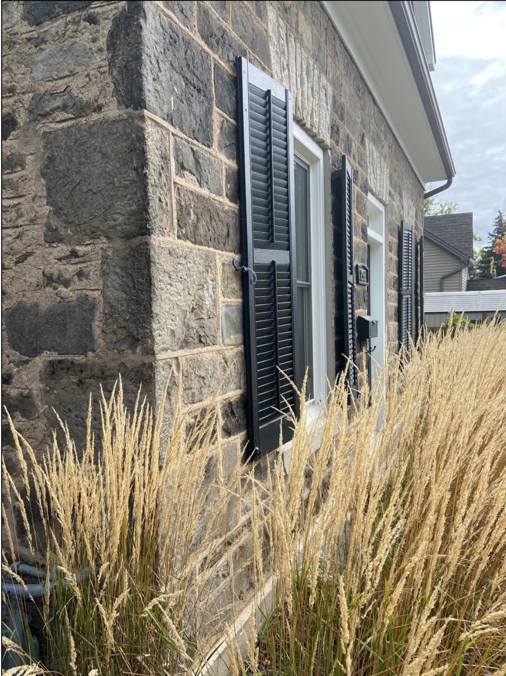
Image 4: Quoin detailing on the façade and western elevations, from the west.
