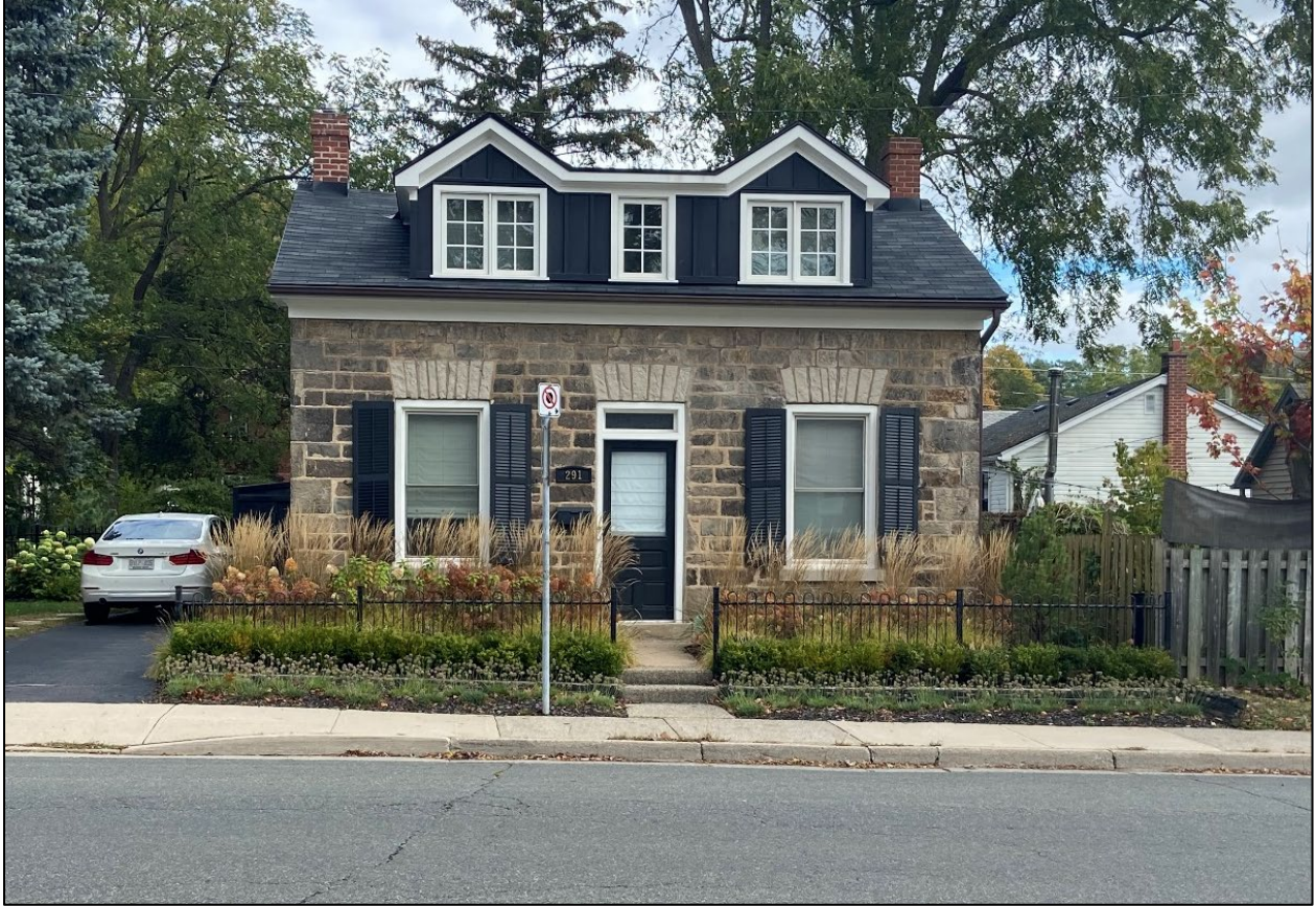
Image 1: Front (southern) elevation, from the south.
