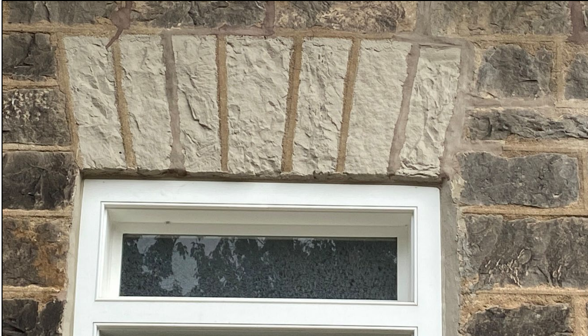
Image 6: Close-up of the front door's transom window and stone voussoir.
