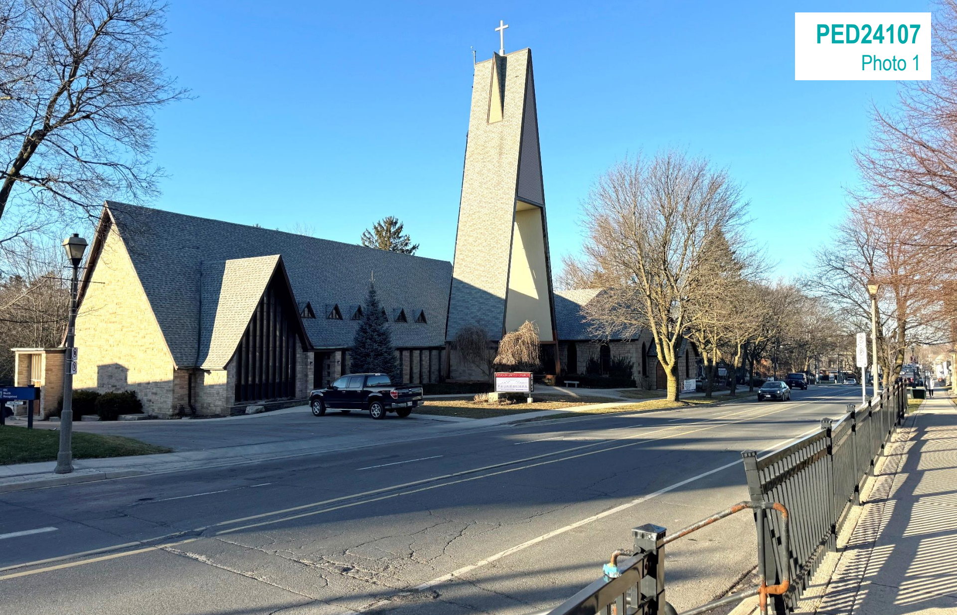
Existing Place of Worship at 265 Wilson Street East, as seen from Wilson Street East looking north east
