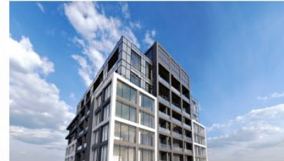
NW VIEW- TOWER TOP
