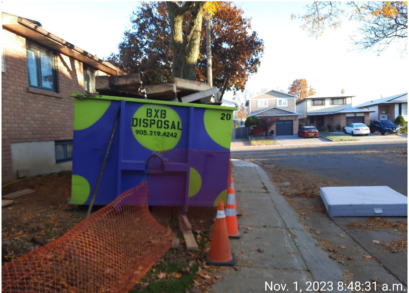
HOMEOWNER BLOCKING SIDEWALK WITH BIN No Road Occupancy Permit
