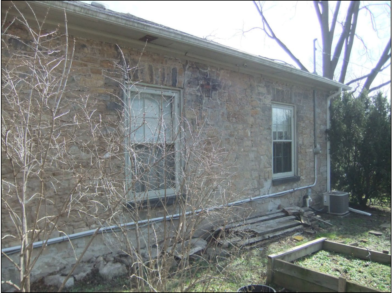
Image 5: Western elevation from a northern vantage point.
