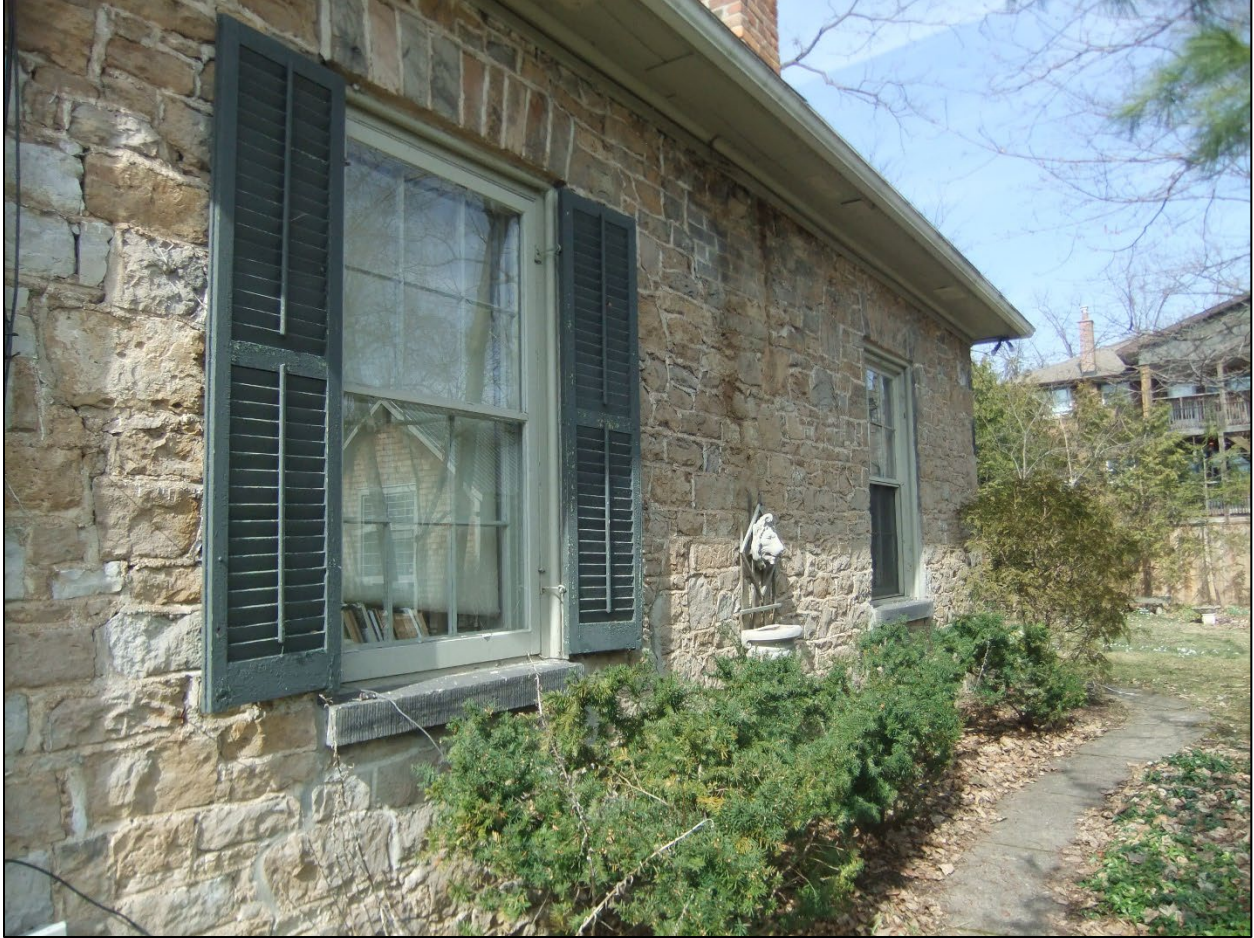
Image 7: Eastern elevation from a southern vantage point.
