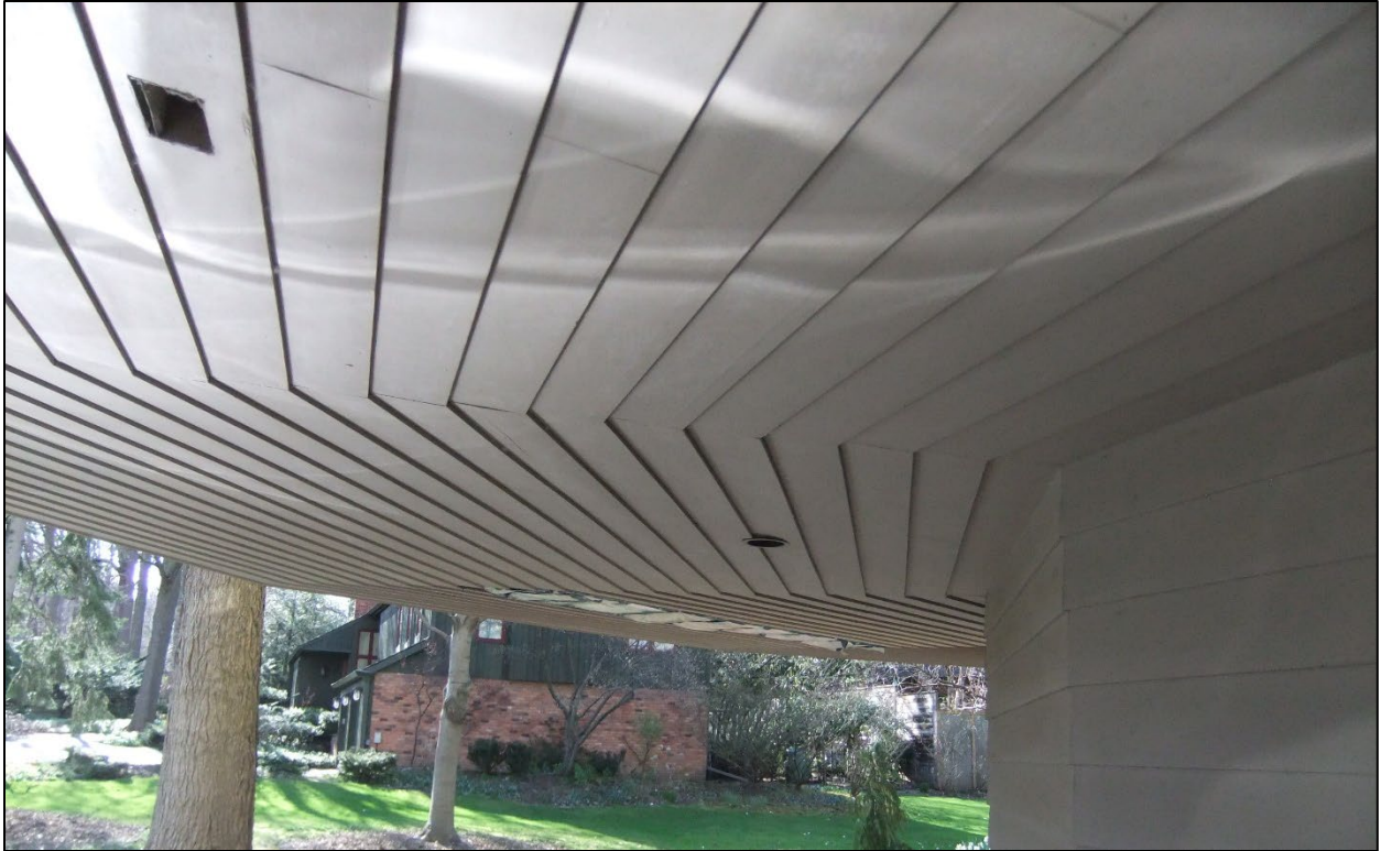
Image 7: Close-up detail of the cedar board cladding underneath the second storey of the Lennard / Mushroom house.
