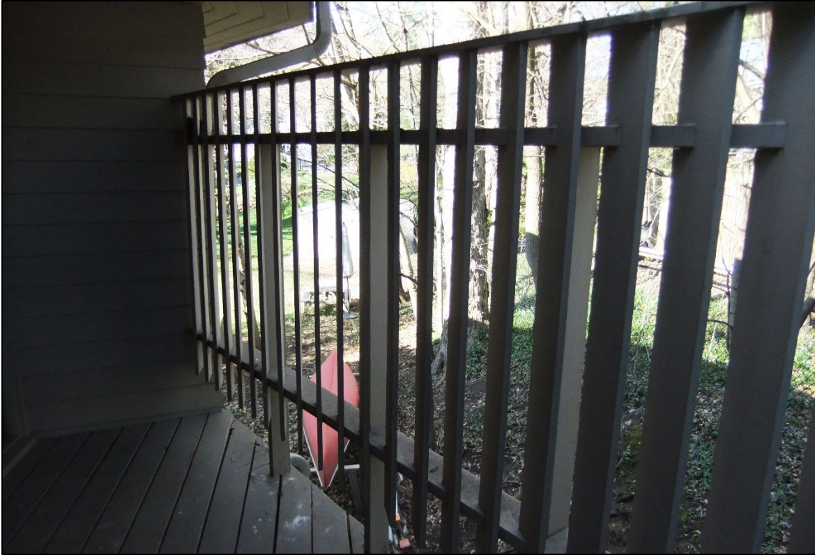
Image 5: Close-up detail of the fence along the second floor entry porch.
