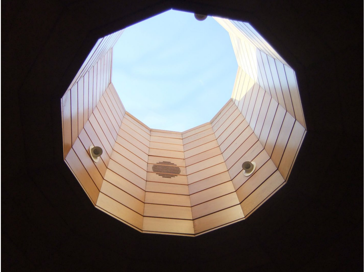
Image 14: Image of the interior portion of the skylight, located centrally in the building, lined with stained cedar.
