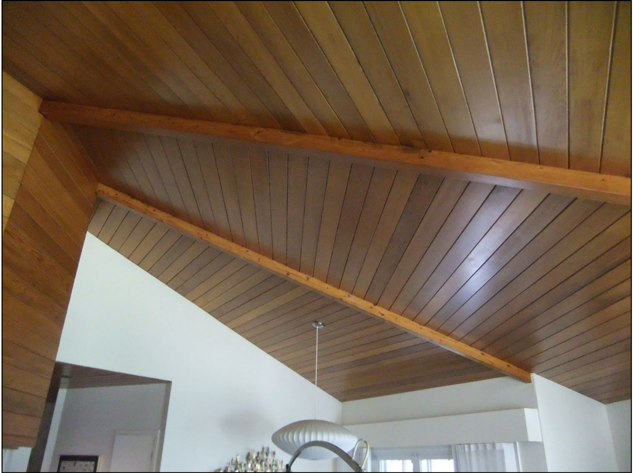
Image 16: Image of the stained cedar ceiling in the main living area, extending to the outer walls.
