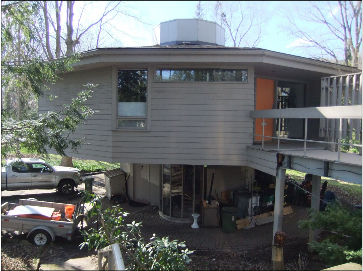
Image 4: Southeastern second storey elevation from the eastern elevated drive and entry way. Note the protected second storey entrance, bridge, and angled decorative fence.
