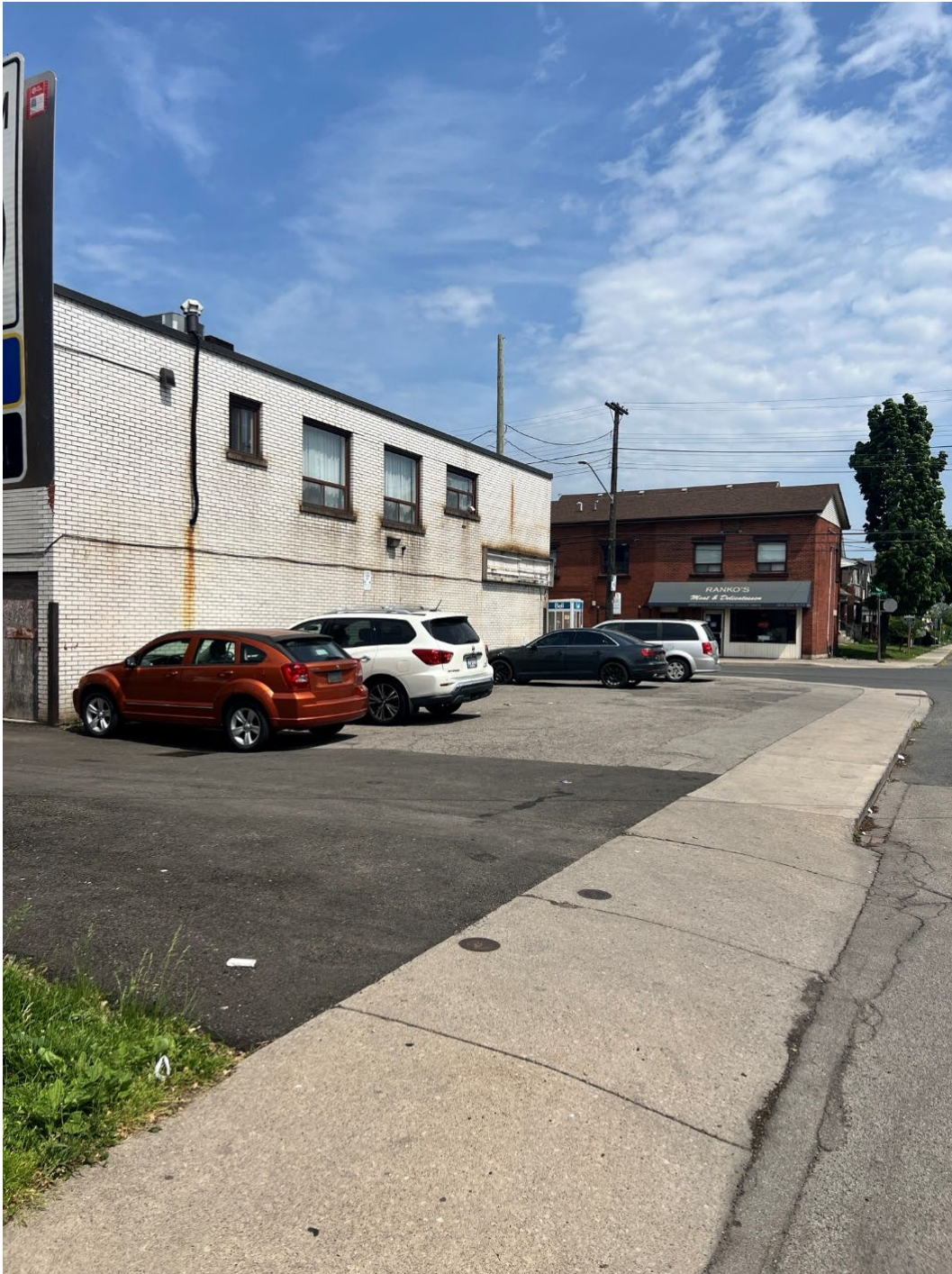
Image 1 - View from southeast corner of the Subject Lands along the frontage on Rosslyn Avenue North looking northwest.
