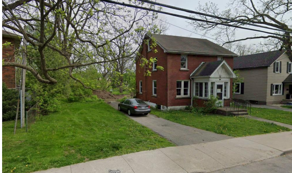
Image Above: Existing 2-1/2 storey brick dwelling at 56 York Rd.
