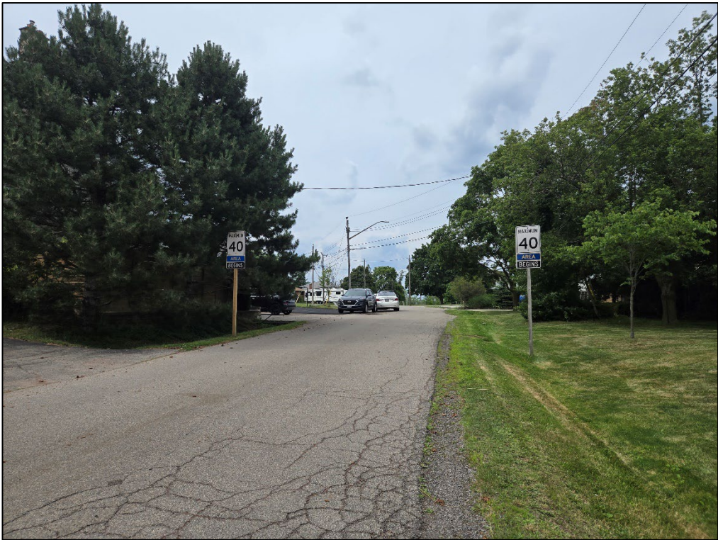
Figure 14 – Millikin Drive at Highway 8 Access – Looking North
