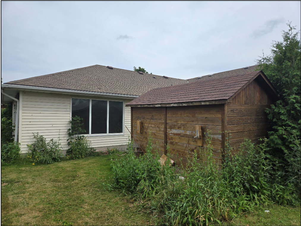
Figure 3 - 1335 Highway 8 – West Side of Dwelling
