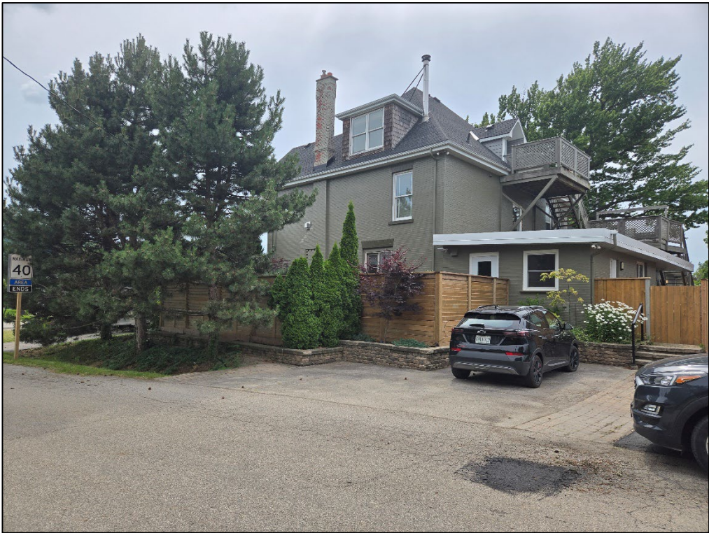
Figure 10 – 1317 Highway 8 – Access from Millikin Drive
