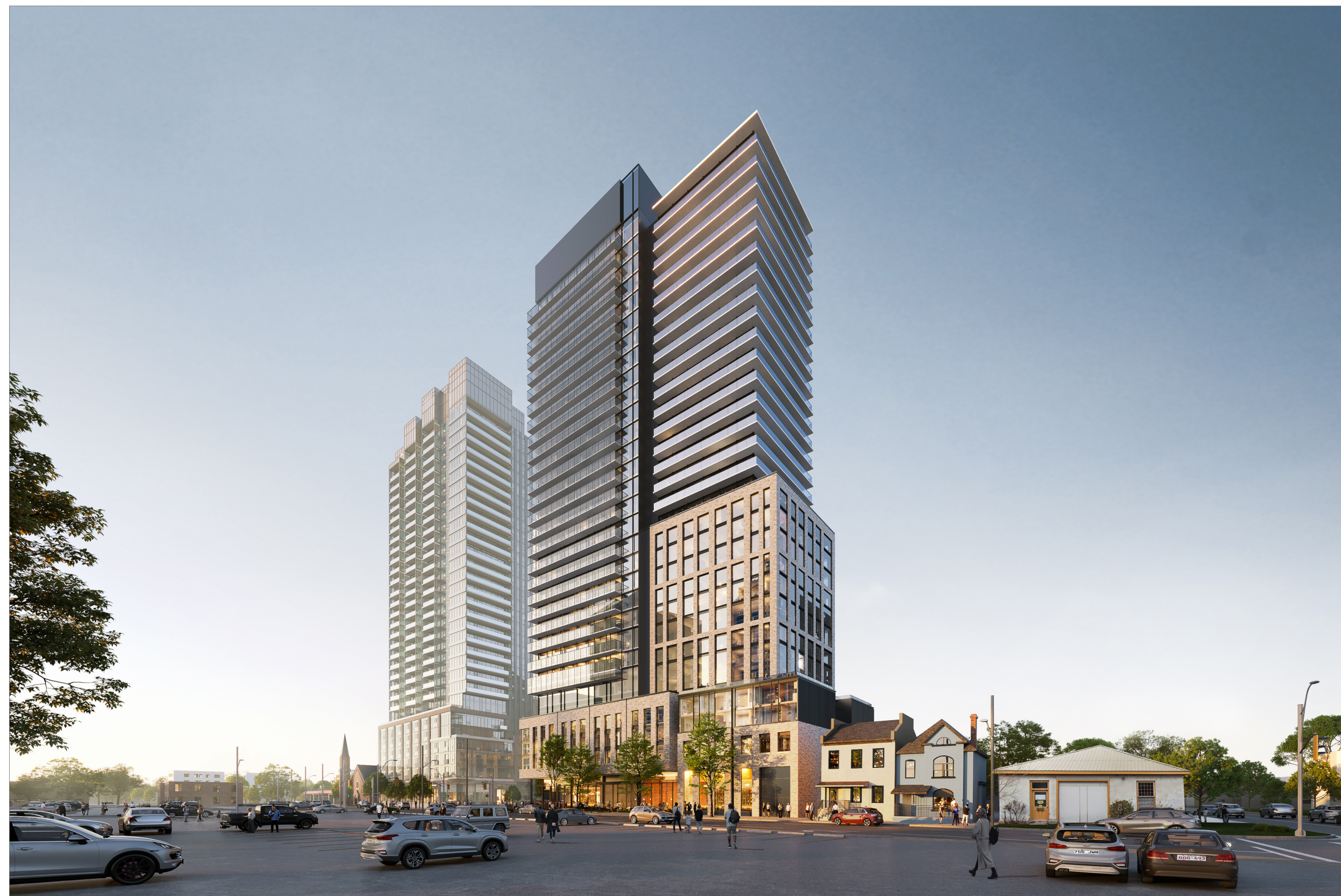
3 VIEW LOOKING AT THE SOUTH EAST CORNER
