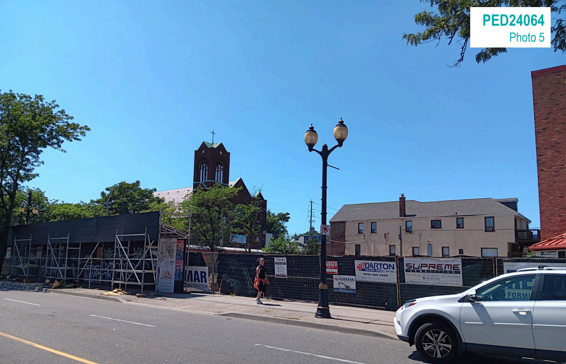
309 James Street North - looking west
