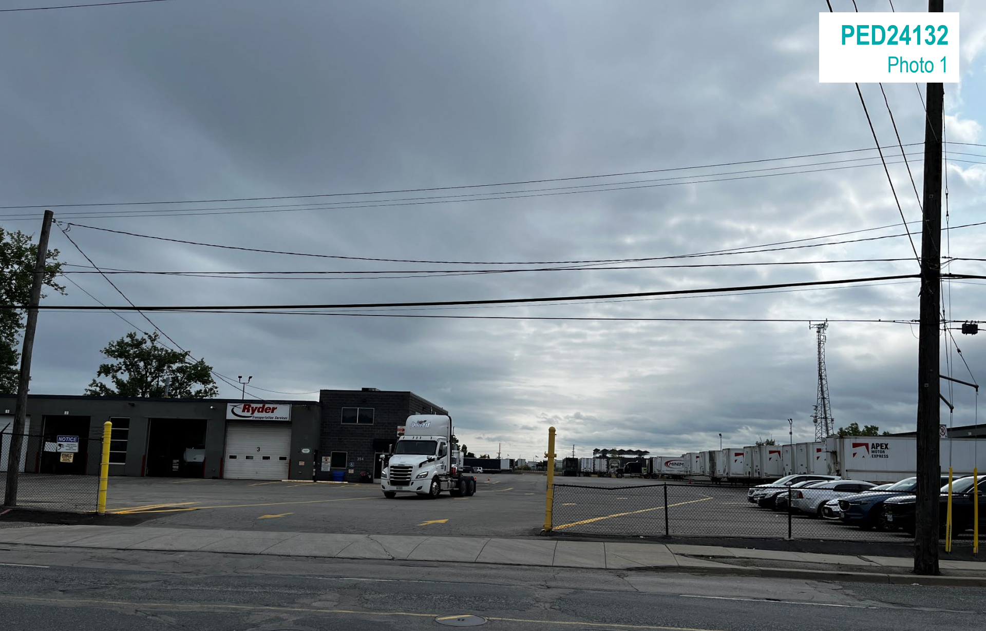
North gate of the Subject Property
