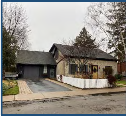
Example of Attached Garage
