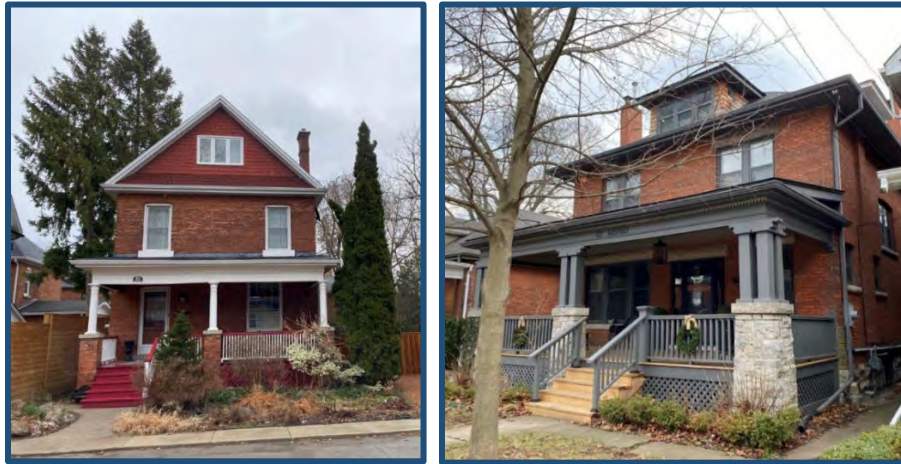
Photos 19 & 20 - (left) Example of Edwardian building located at 31 Princess Street, c. 1916 (right) Example of Edwardian building influenced by the American Four-Square architectural style, located at 122 Melville Street, c. 1904 (Source: MHBC, 2023)
