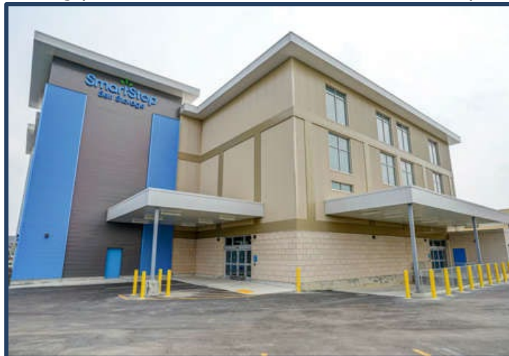
Figure 38: Enhanced secondary façade of 60 Cityview Boulevard, Vaughan (Source: SmartStop Self Storage)
