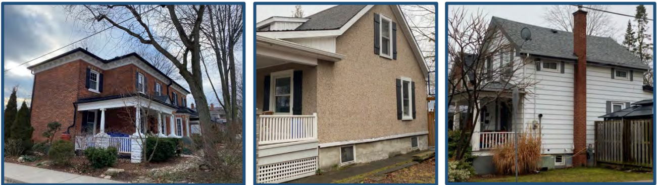
Photos 30-32 - (left) Example of a red brick dwelling; (middle) Example of a pebbledash stucco clad building; (right) Example of a building clad with synthetic siding (Source: MHBC, 2023)
