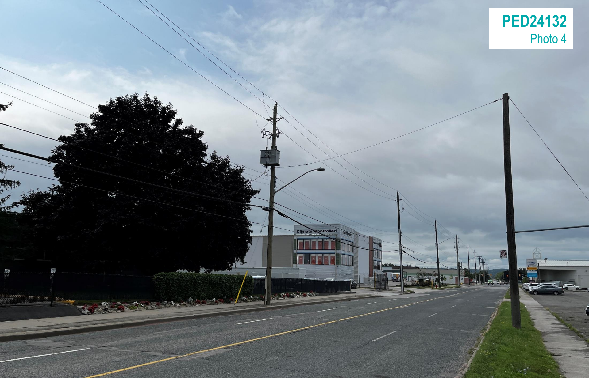
Nash Road North looking south
