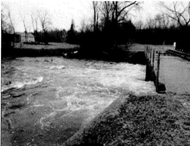
Photo 55 Downstream View of Bennett Dam
