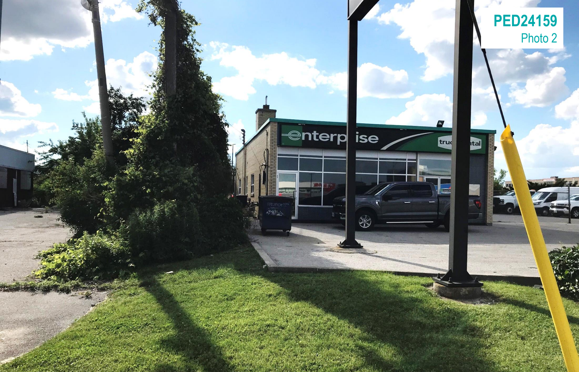
Adjacent commercial building to the north
