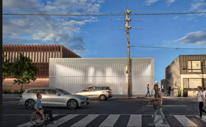
EXAMPLE: TRACTION POWER SUBSTATION PAPE AND SAMMON AVENUE, TORONTO
