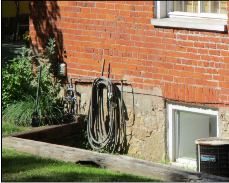
Image 17: Detail of stone foundation on south elevation.
