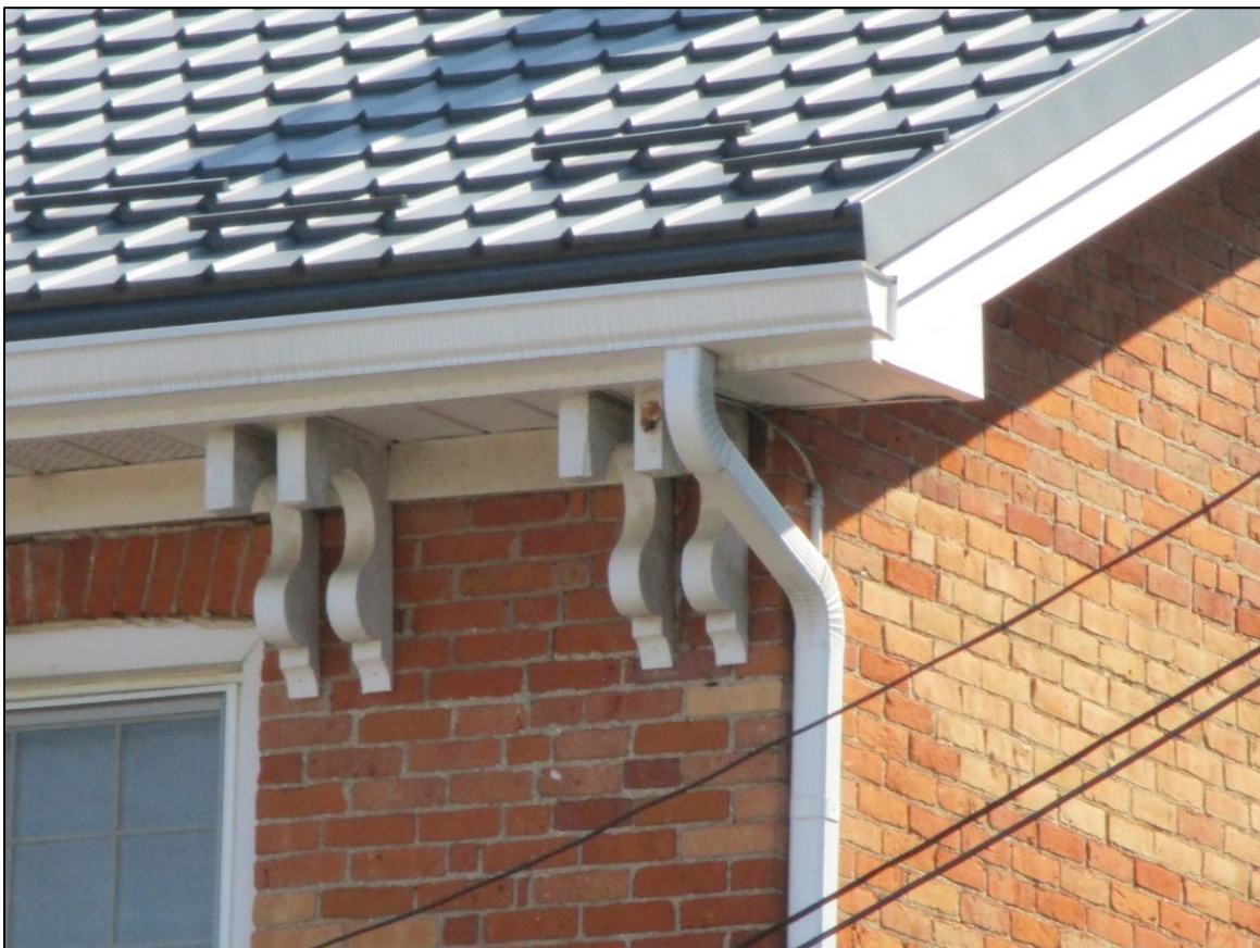
Image 10: Detail of brackets on western end of the north elevation of the rear wing.
