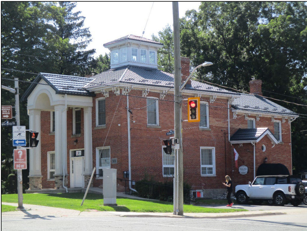
Image 2: Orton House, looking southwest from the intersection of Wilson Street East and Sulphur Springs Road.
