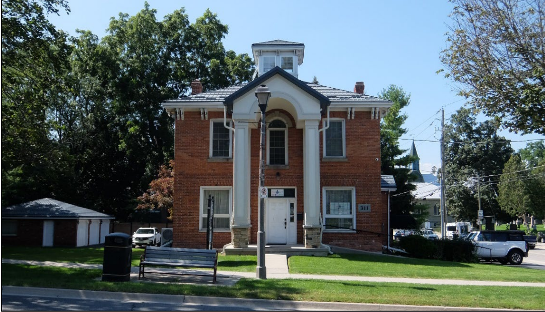
Image 1: Front (east) elevation of property.
