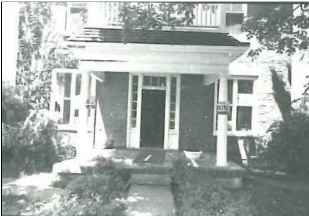
Image 28: Detail of front balcony and entrance, circa 1977 (Ancaster LACAC).
