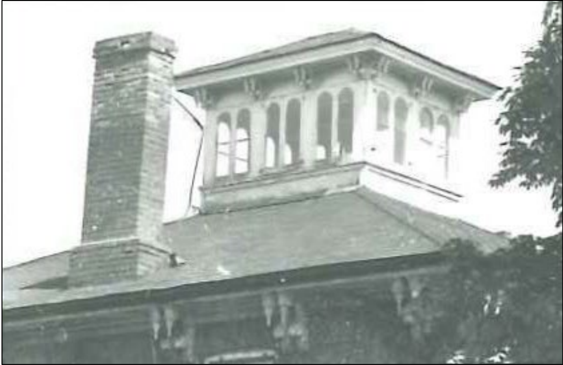
Image 27: Detail of belvedere and chimney, circa 1977 (Ancaster LACAC).
