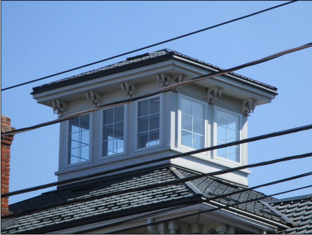
Image 7: Detail of belvedere looking south.
