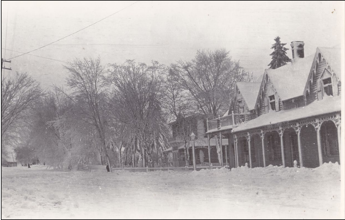
Image 30: Wilson Street looking southbound, late-nineteenth century. Subject property in center. (Hamilton Public Library, Local History and Archives).
