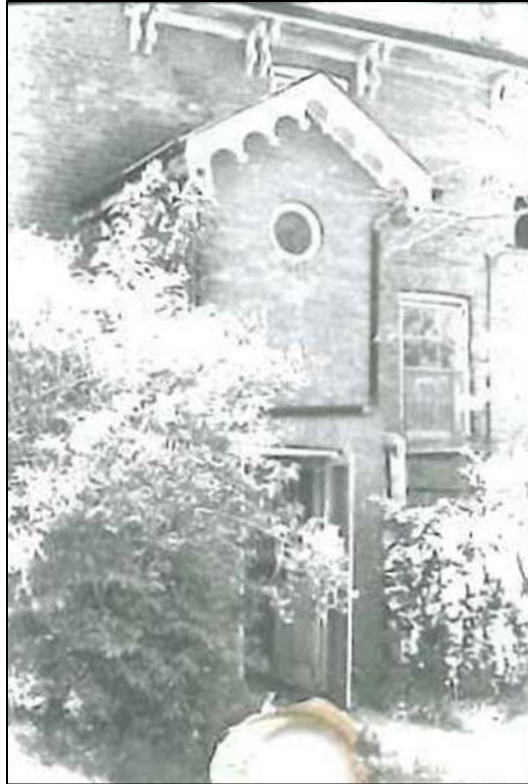
Image 23: Detail of side entrance, circa 1977, showing former bargeboard detail in the projecting gable (Ancaster LACAC).
