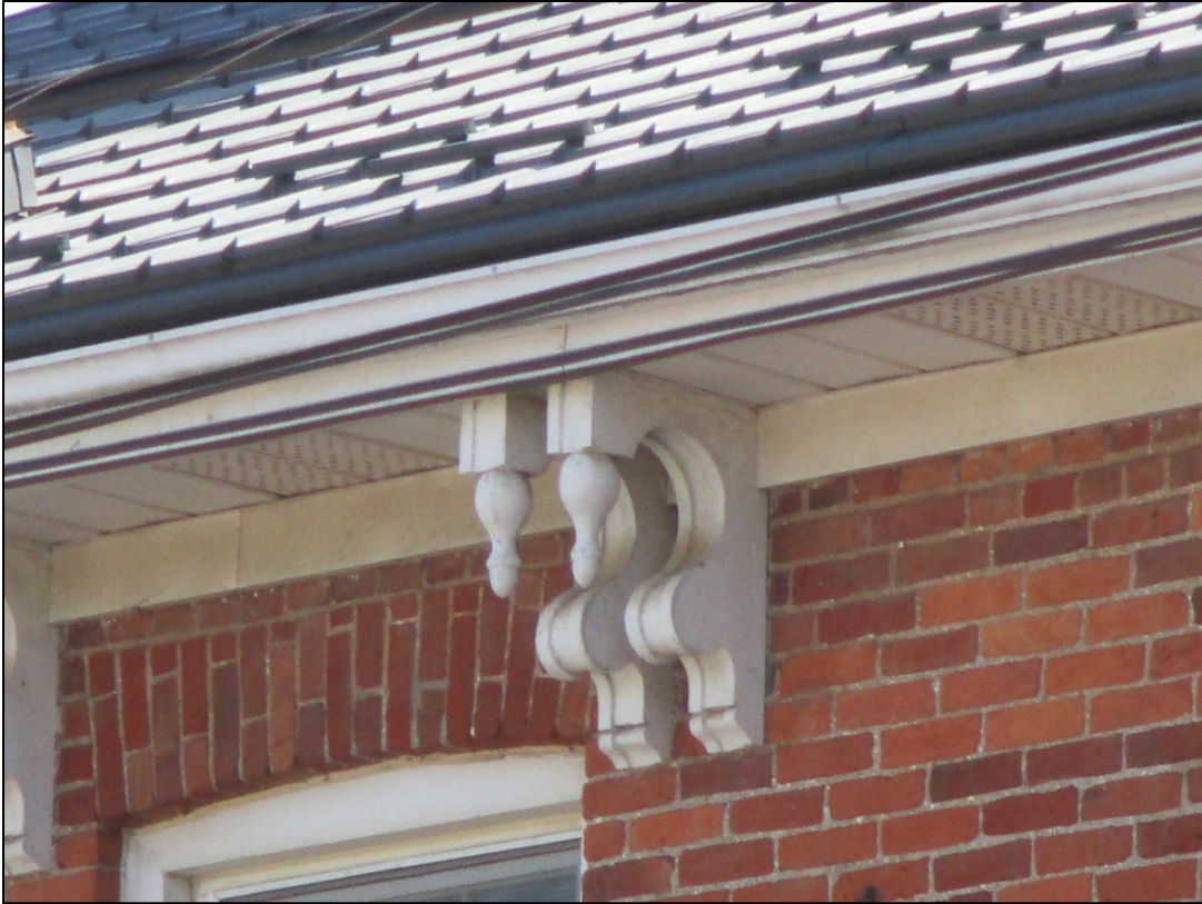
Image 11: Detail of brackets on the eastern end of the north elevation.
