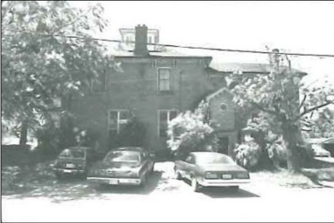
Image 19: North elevation looking from Sulphur Springs Road, circa 1977 (Ancaster LACAC).
