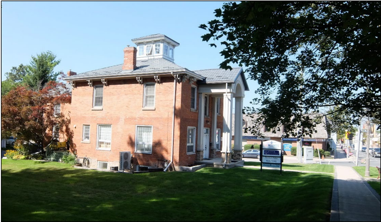
Image 3: South elevation, looking north up Wilson Street East.
