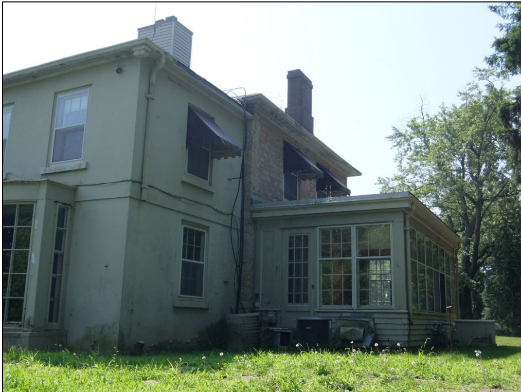
Figure 4: View of northeastern corner of property.
