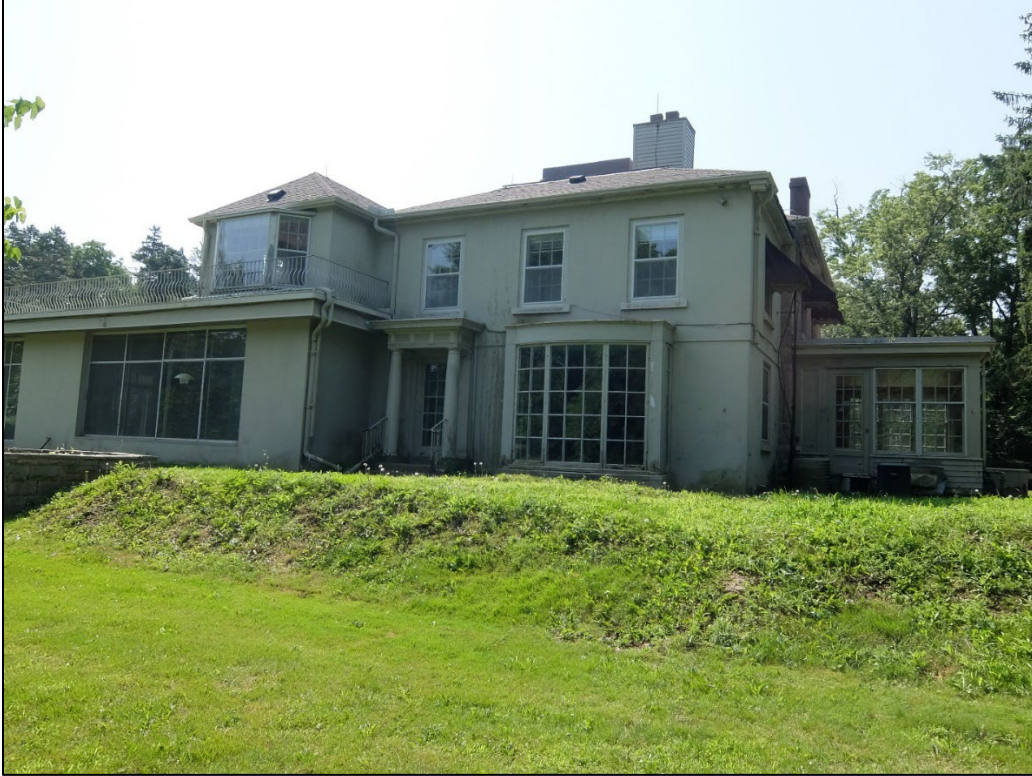
Figure 5: View of northern (rear) elevation.
