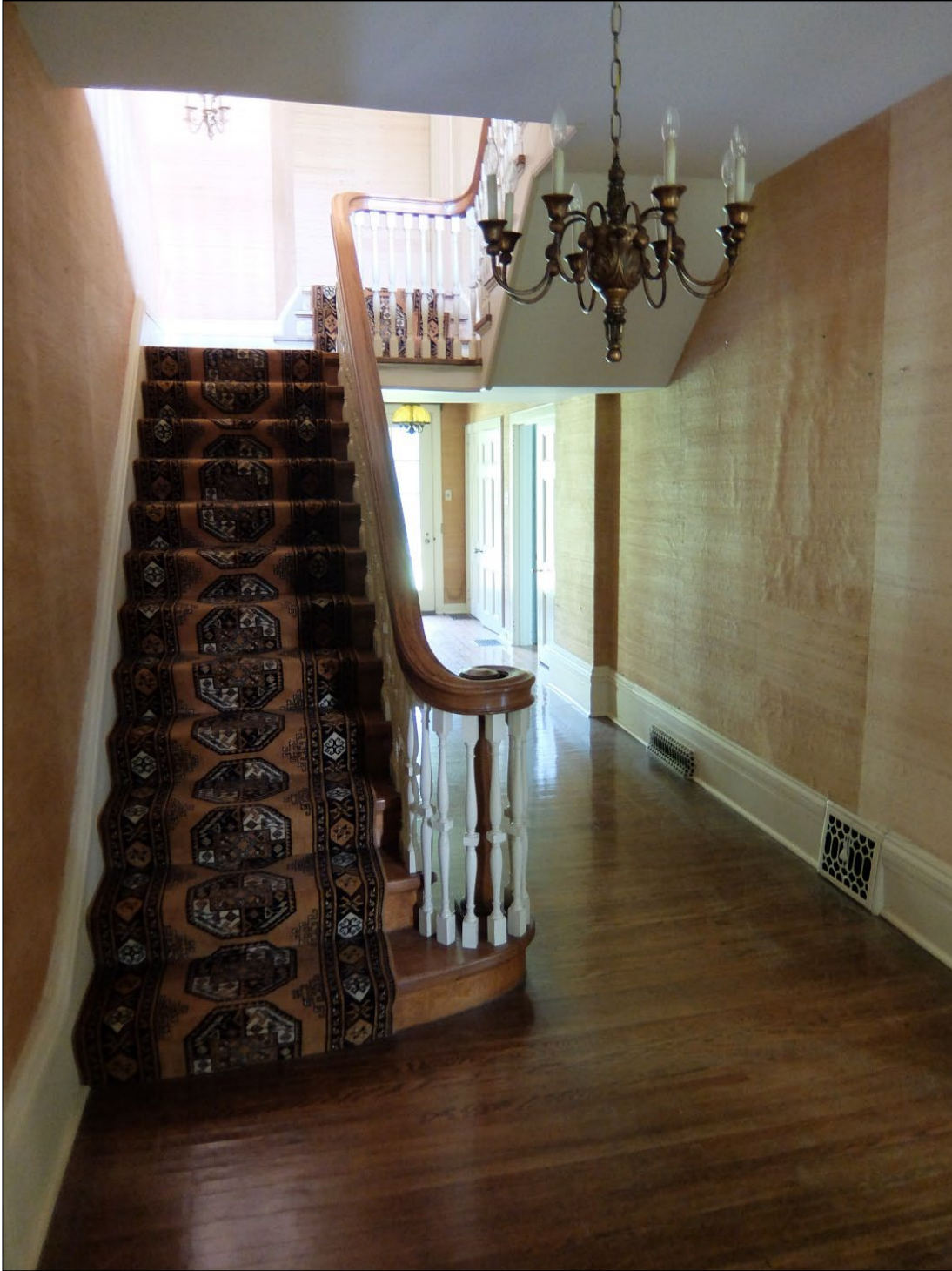
Figure 16: Interior view of property, showing central quarter-sawn American white oak staircase.
