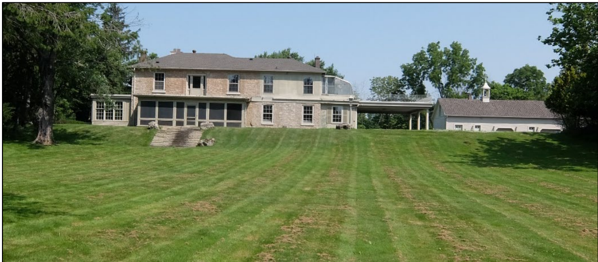
Figure 2: View of south (front) elevation of the building, showing the original circa 1846 Neoclassical residential building to the left, side additions with covered drive and detached accessory building.
