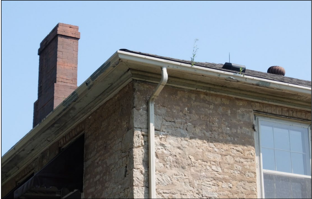
Figure 9: Detail view of eaves showing cornice.
