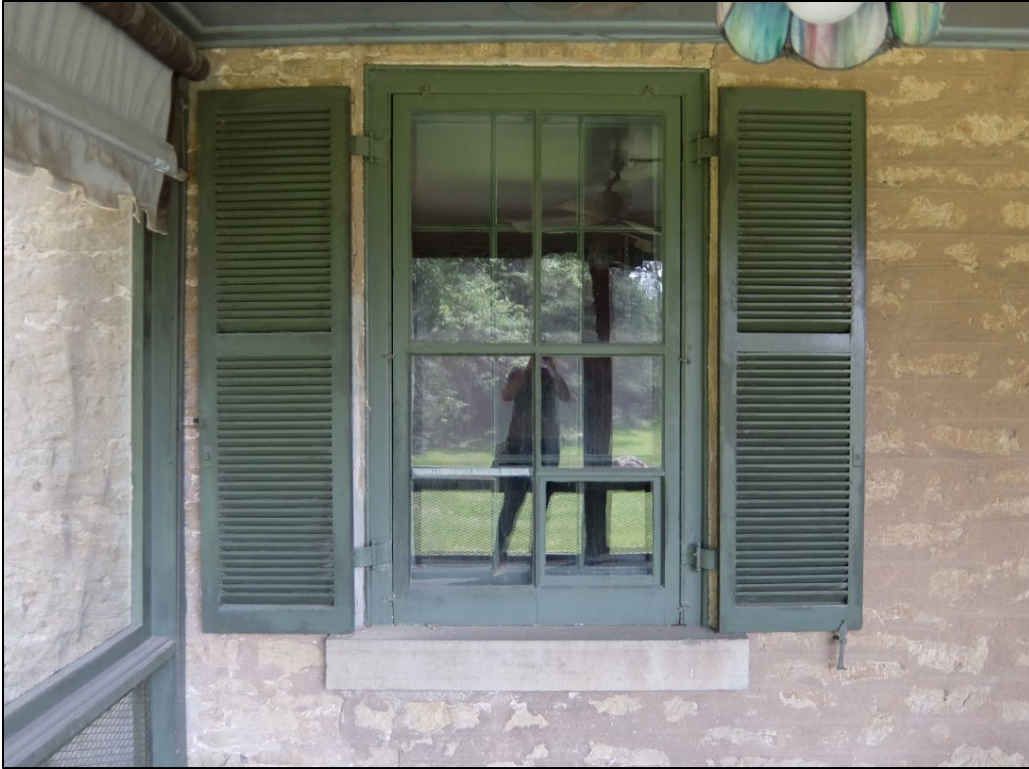
Figure 11: Detail view of window on south elevation showing wooden storms and shutters and stone sill.
