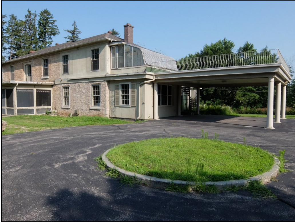
Figure 7: View of southwestern elevation showing side additions.
