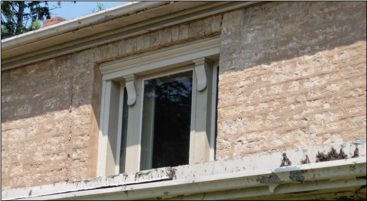
Figure 13: Detail view of Venetian window on south (front) elevation.
