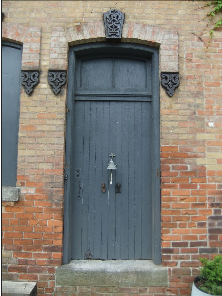
Image 3: Close-up of the eastern elevation door.
