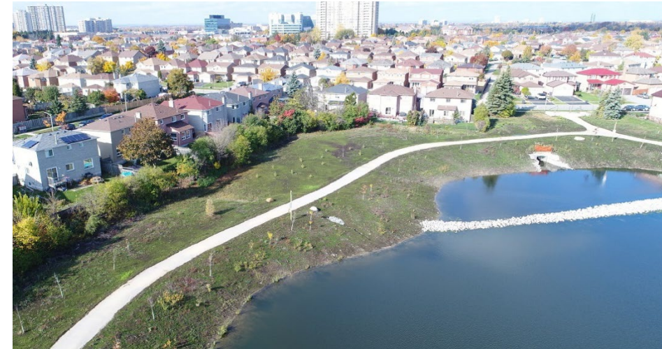
Extended Detention Wet Pond Example (ref. TRCA, 2020)
