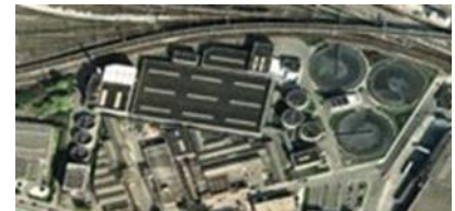
Brussels Sud WWTP, Belgium ADF 86 MLD (23 MGD) MDF 190 MLD (44 MGD) Commissioned 2018
