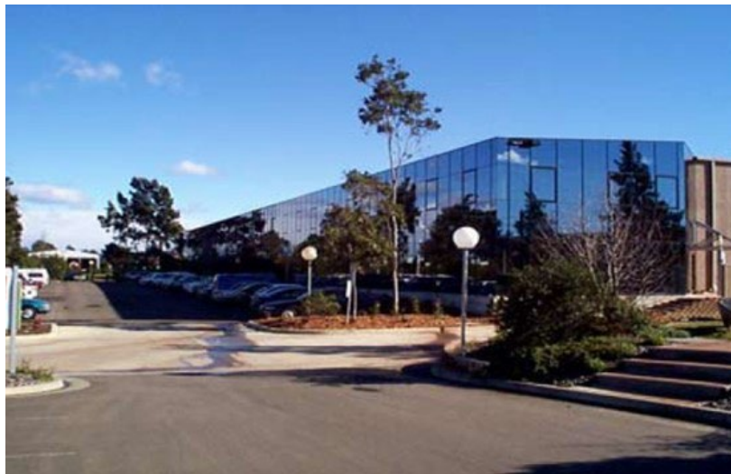
MEMCOR Facility in Windsor, New South Wales, Australia
