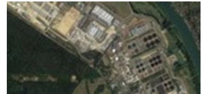
Seine Aval WWTP, France ADF 218 MLD (59 MGD) MDF 348 MLD (92 MGD) Commissioned 2017
