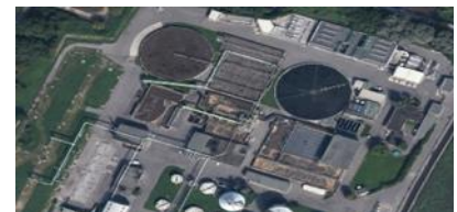
Brescia WWTP, Italy ADF 30 MLD (8 MGD) MDF 60 MLD (16 MGD) Commissioned 2002 Proven membrane life 14 years
