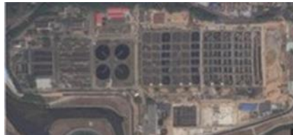
Luo Fang WWTP, China ADF 400 MLD (106 MGD) MDF 462 MLD (122 MGD) Commissioned 2018
