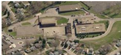
Euclid WWTF, USA ADF 83 MLD (22 MGD) MDF 250 MLD (66 MGD) Commissioned 2018
