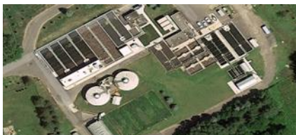
Oxford WWTP, Canada ADF 13 MLD (3.6 MGD) MDF 25 MLD (6.8 MGD) Commissioned 2008 Proven membrane life 14 years
