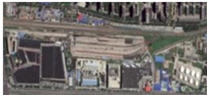
Beijing Shunyi WWTP, China ADF 180 MLD (48 MGD) MDF 234 MLD (62 MGD) Commissioned 2016
