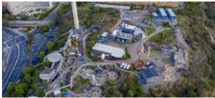
Henriksdal WWTP, Sweden ADF 536 MLD (142 MGD) MDF 864 MLD (228 MGD) PH1 Commissioned 2020
