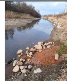
Note 1: Kay Dredge Park Storm Pipe
