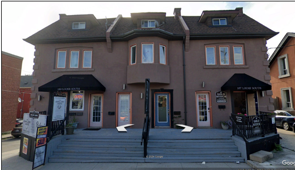
Figure 2: Locke Street South Facade.
