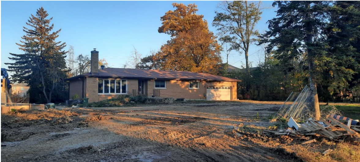
Photo 1: Subject Lands Facing East from Springbrook Avenue
